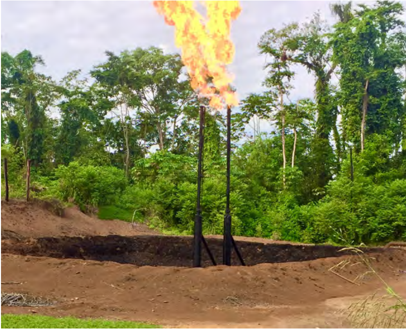
FIGURE 33 The massive gas flares popularly called “el dragón” at the Drago Norte-1 station. Photo by author.
