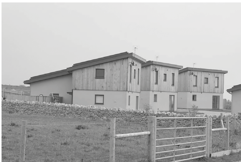
Figure 4.5 Sustainable homes at Worth Matravers, Dorset. © ARCO2.
