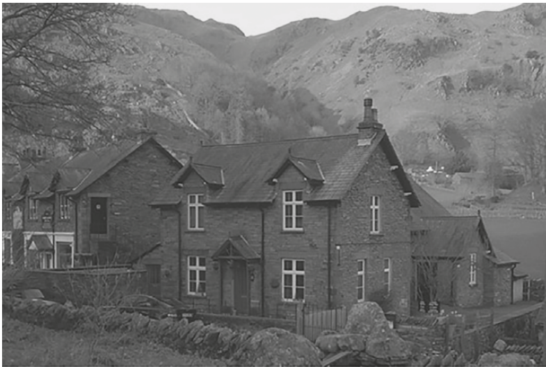
Figure 4.3 Church Hall Cottage, Chapel Stile, Lake District. © Skelwith and Langdale CLT.
