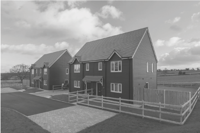
Figure 4.2 Little Stocks Close, Kinlet, Shropshire. © Shropshire Rural HA.
