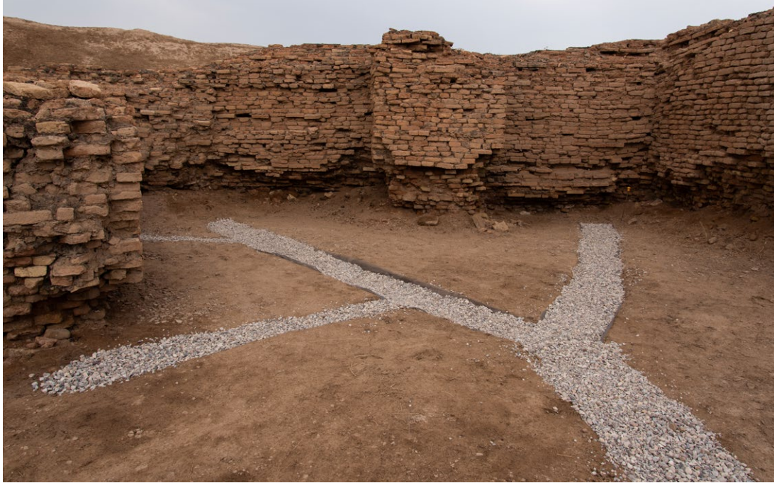
Figure 26.7 Drainage channels installed to drain off water from the bridge at Tello
