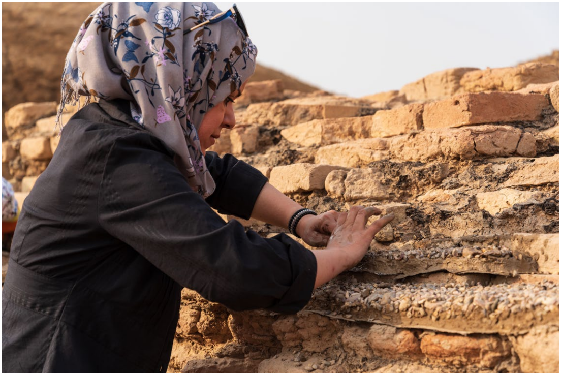
Figure 26.4 Restoration of the third millennium bridge at Tello
