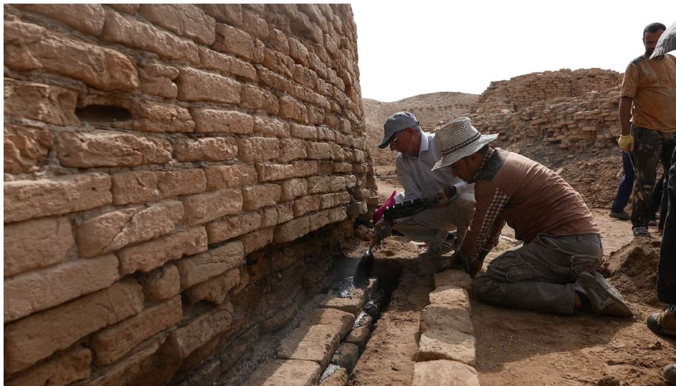
Figure 26.9 Repairing the foundations of the bridge at Tello
