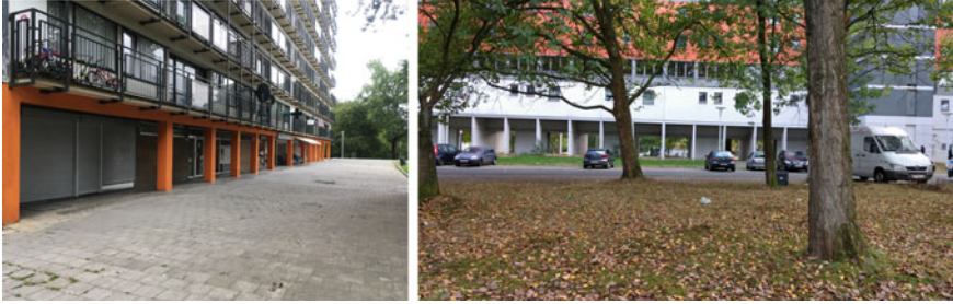
Fig. 13.1 The architecture of the ground floors in Peterbos
