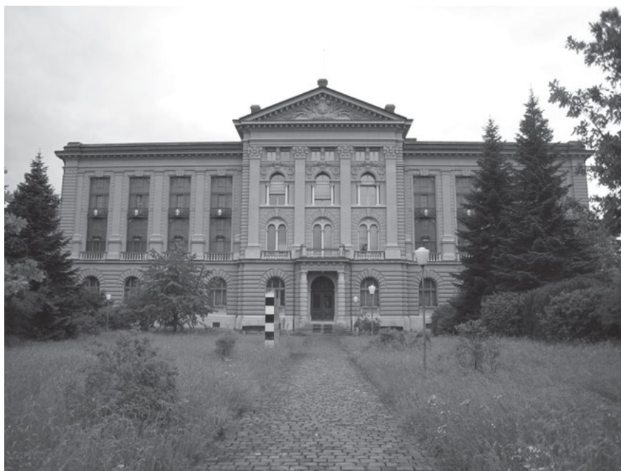
Figure 11.1: Federal Archives of Switzerland in Berne, completed in 1899.
