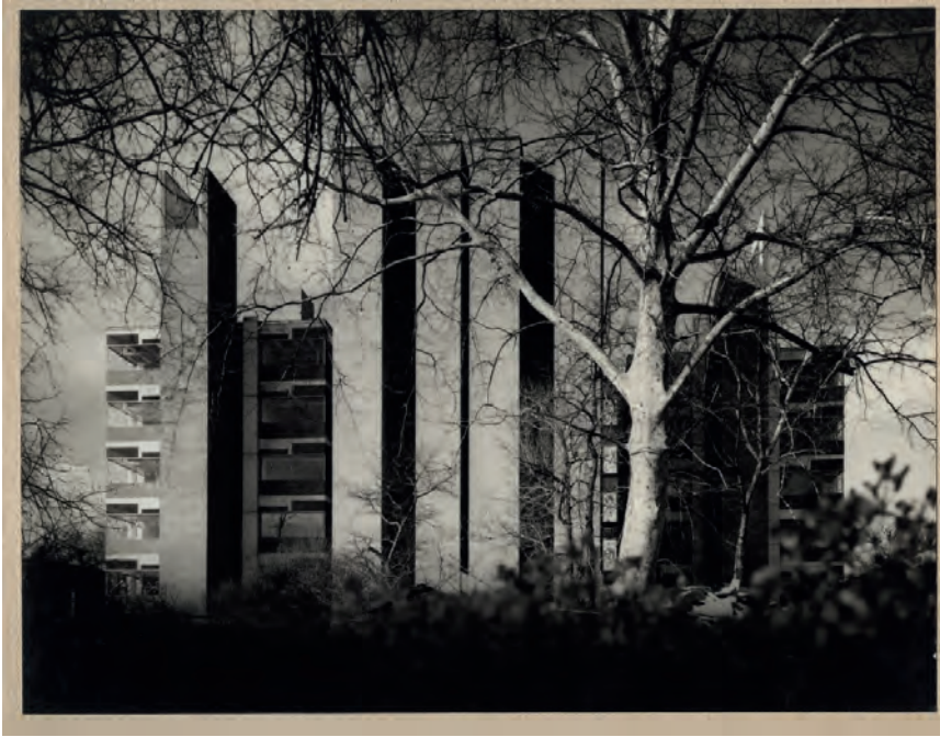
Fig. 101: Louis I. Kahn, Alfred Newton Richards Medical Research and David Goddard Laboratories Buildings, University of Pennsylvania, Philadelphia, 1957-65.
