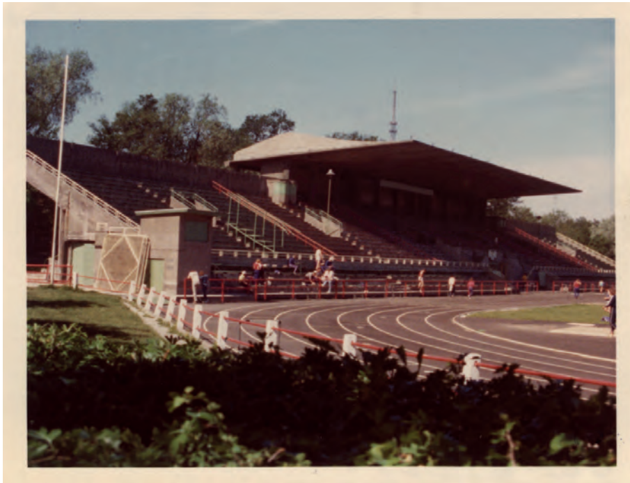
Fig. 110: August E. Komendant, Tribune Kadrioru Stadium, Tallin, Estonia, 1936-7.
