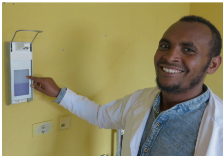
Hand sanitizer dispensers are installed throughout the hospital
