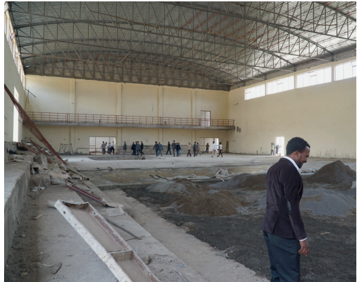
The gymnasium of Arsi University under construction
