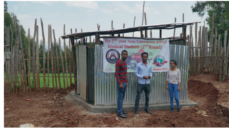
Newly-built toilets on the marketplace of a small town near Asella
