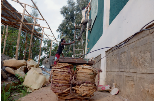
In Ethiopia, you have to be able to improvise with the tools – like with this welder
