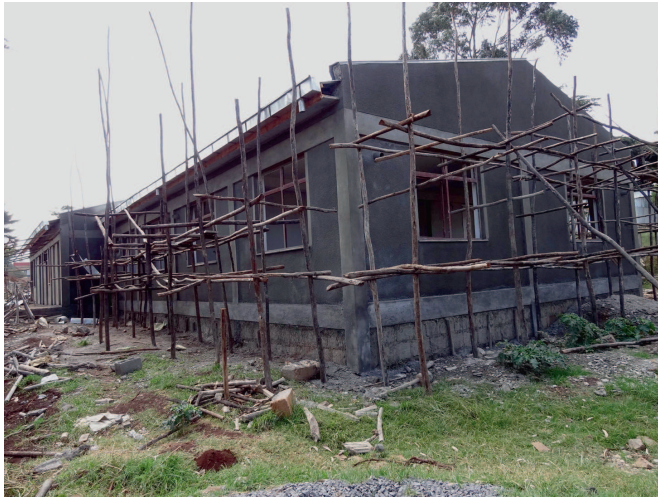
The shell of the Hirsch Institute surrounded by traditional scaffolding in 2011
