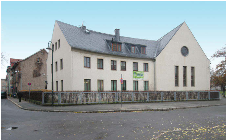
Fig. 3: Erfurt Synagogue, view from north-east (Photograph: Ulrich Knufinke, Bet Tfila – Research Unit for Jewish Architecture, Braunschweig, 2008).
