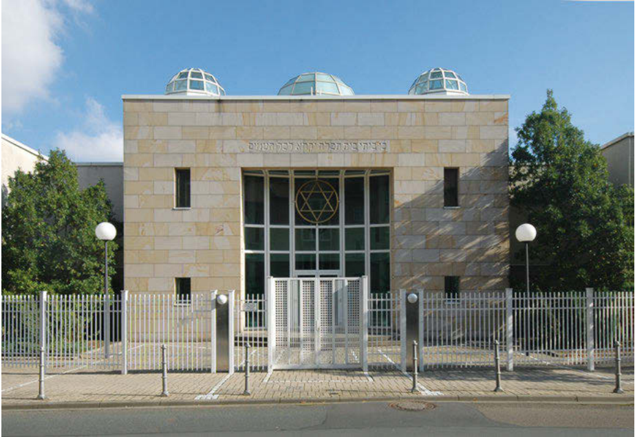
Fig. 5: Darmstadt Synagogue (1988), façade from west (Photograph: Ulrich Knufinke, Bet Tfila – Research Unit for Jewish Architecture, Braunschweig, 2007).
