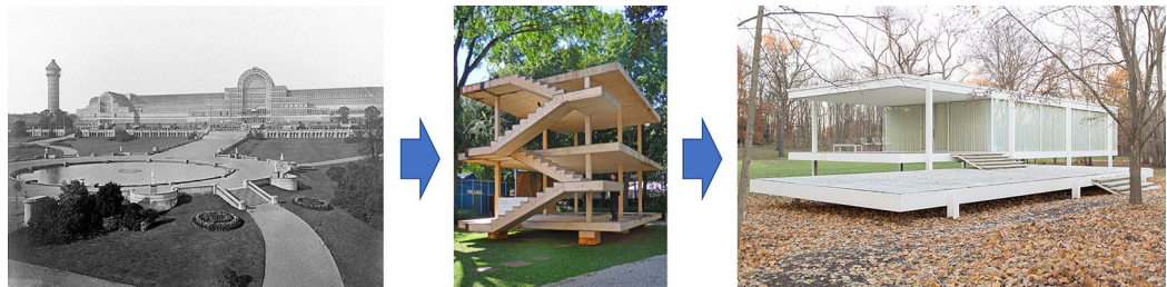
Fig. 02. The rebuilt Christal Palace at Sydenham in 1930 (left– public domain image), the Dom-ino house by Le Corbusier (1914) rebuilt for the Biennale of Architecture in Venice in 2014 (centre – public domain image). These iconic buildings are part of the process that led to contemporary glass house.
