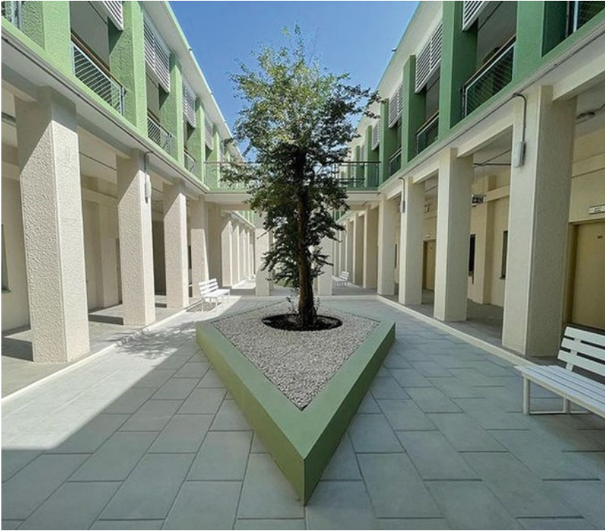
Fig. 14.9 Liwan building, by Qatar Museums (Qatar Museums)
