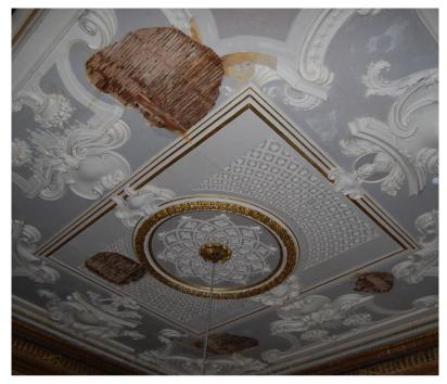
**Figure 1.18:** Clandon Park, the Speakers' Parlour ceiling in the days after the fire, showing its remarkable survival. © National Trust Images/John Millar.
