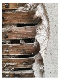
**Figure 1.30:** Layers revealed by the fire, including the softwood laths and three layers of plaster.
