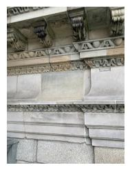
**Figure 8.4:** Old Library, Trinity College Dublin. Cornice-level carvings in Scrabo sandstone (top), Calp limestone (middle) and ashlar granite (bottom). Compared with contemporary carvings in Portland stone in Dublin these are rather crude. Some of the sandstone has been replaced with moulded mortar.
