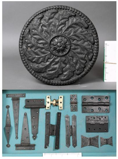
**Figure 3.29:** (a) Cast-iron coal-hole cover, South Frederick Street, Dublin, mid-eighteenth century; (b) eighteenth-century hinges, including shutter hinges.
