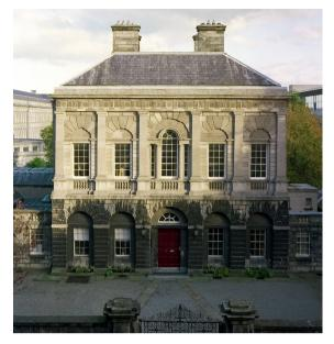
**Figure 8.13:** Ardbraccan limestone, Provost's House, Trinity College Dublin. The icicle rustication on the ground floor has allowed for the build-up of soot and gypsum while the upper story, being plain ashlar, remains cleaner. Photograph by Stephen Farrell.
