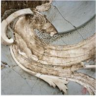
**Figure 9.8:** Early eighteenthcentury plasterwork where sections of the applied ornament have fallen away to reveal the scored surface underneath in the dirty white central section. Small parts of the modelled leaf have survived around the edges of the exposed scoring. © Richard Ireland.
