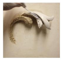
**Figure 9.22:** Lime-plaster modelling demonstration. © Jenny Saunt.
