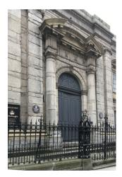
**Figure 8.5:** St Werburgh's Church, Dublin. Entrance façade with Calp limestone plinth and worked Scrabo sandstone laid in a pattern of courses of unequal size.
