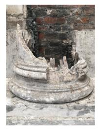
**Figure 1.28:** An engaged column in the Marble Hall: partially burned, it reveals the timber structure beneath the plaster.
