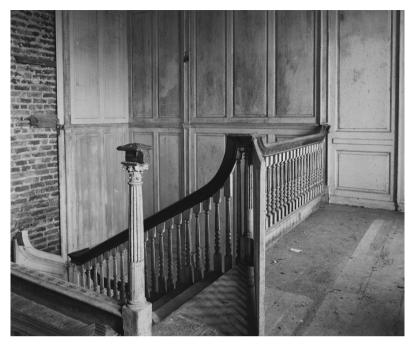
**Figure 3.10:** Former staircase, showing newel post, Kilmacurragh, County Wicklow, built circa 1697–1705.
