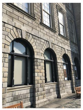
**Figure 8.2:** Calp limestone arcade, Old Library, Trinity College Dublin. The dark muddy limestone on the ground floor offers a visual contrast to the paler granite of the upper storeys.
