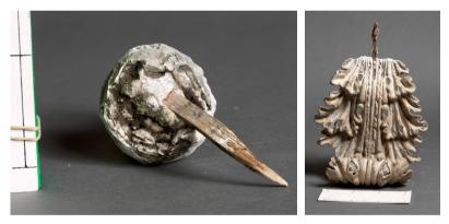
**Figure 3.20:** (a) Peach plaster fragment, showing timber armature, No. 129 St Stephen's Green, Dublin; (b) acanthus leaf, showing nail armature, entrance hall ceiling rose, South Frederick Street, Dublin.
