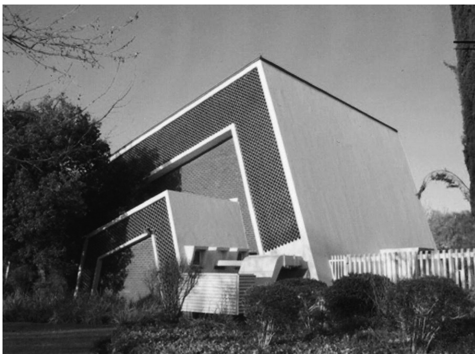
Figure 1.5: The Potchefstroom Conservatory during the 1960s 14
