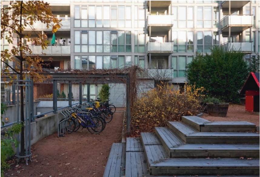
Fig. 3.1 Klosterenga facade seen from the garden. Note: Photo by GASA Architects
