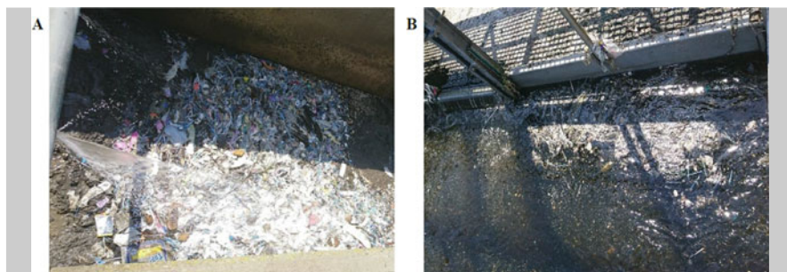
Image 2.1 Evidence of debris in the a dissolved air flotation tank and b effluent of a Cape Town WWTP (Chitaka, 2020)
