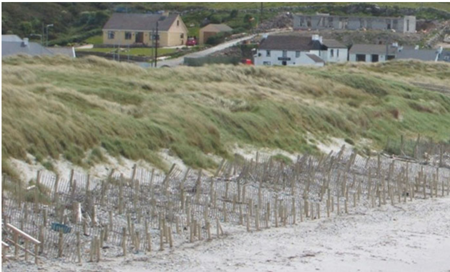
Fig. 32.3 The sand trapping scheme in Maghery in 2006 which was comprised of a lattice network of fencing. (Photo: Prof. Derek Jackson)
