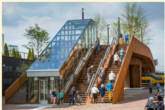
The bridge is accessed via stairs with narrow bicycle ramps and inclined elevators.
