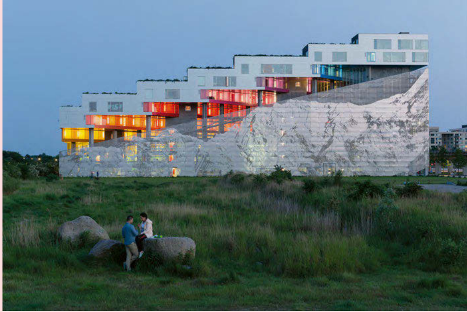
..... The parking garage is framed by a perforated metal façade with a mountain motif. .....
