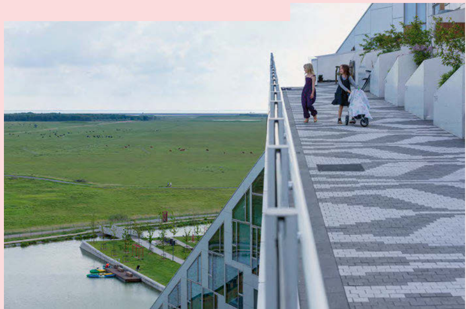
The public path winds once all the way around 8 House up to the top floor.
