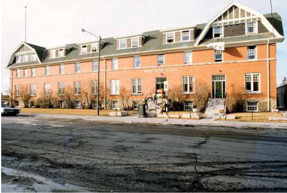
The original Mount Royal College building in downtown Calgary, ca. 1969. The building was demolished shortly after opening of the Lincoln Park Campus in 1972. Mount Royal University Archives G1102.
