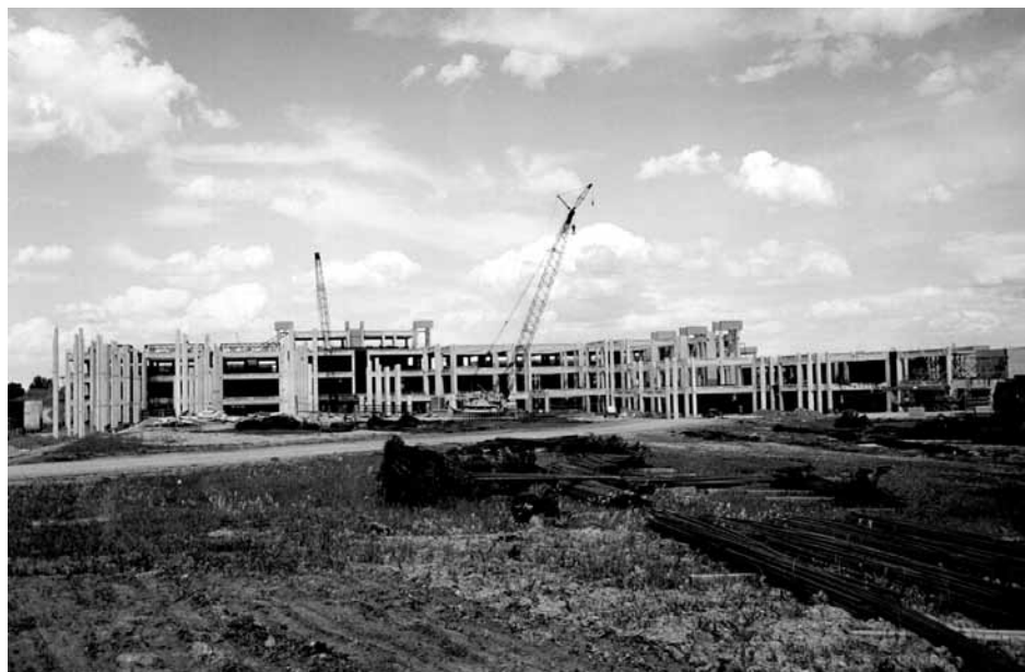
Construction underway on the Lincoln Park Campus, 1971. Photographer Hillhurst Studio; Mount Royal University Archives HB83-2.
