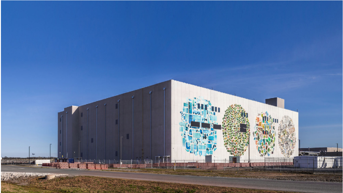
Figure 4.1: Google’s four-story cloud data center in Mayes County, Oklahoma.
