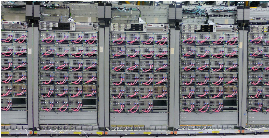
Figure 3.7: Interconnected GPUs for training.
