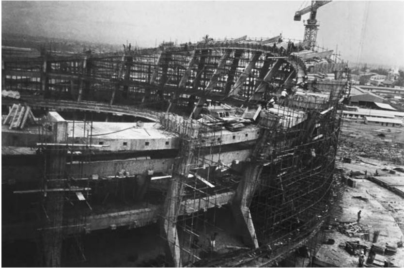
FIGURE 34. National Theatre in Lagos, construction in progress. Source: TsDA, f. 608, op. 6P, a.e. 6, Technoexportstroy catalog.
