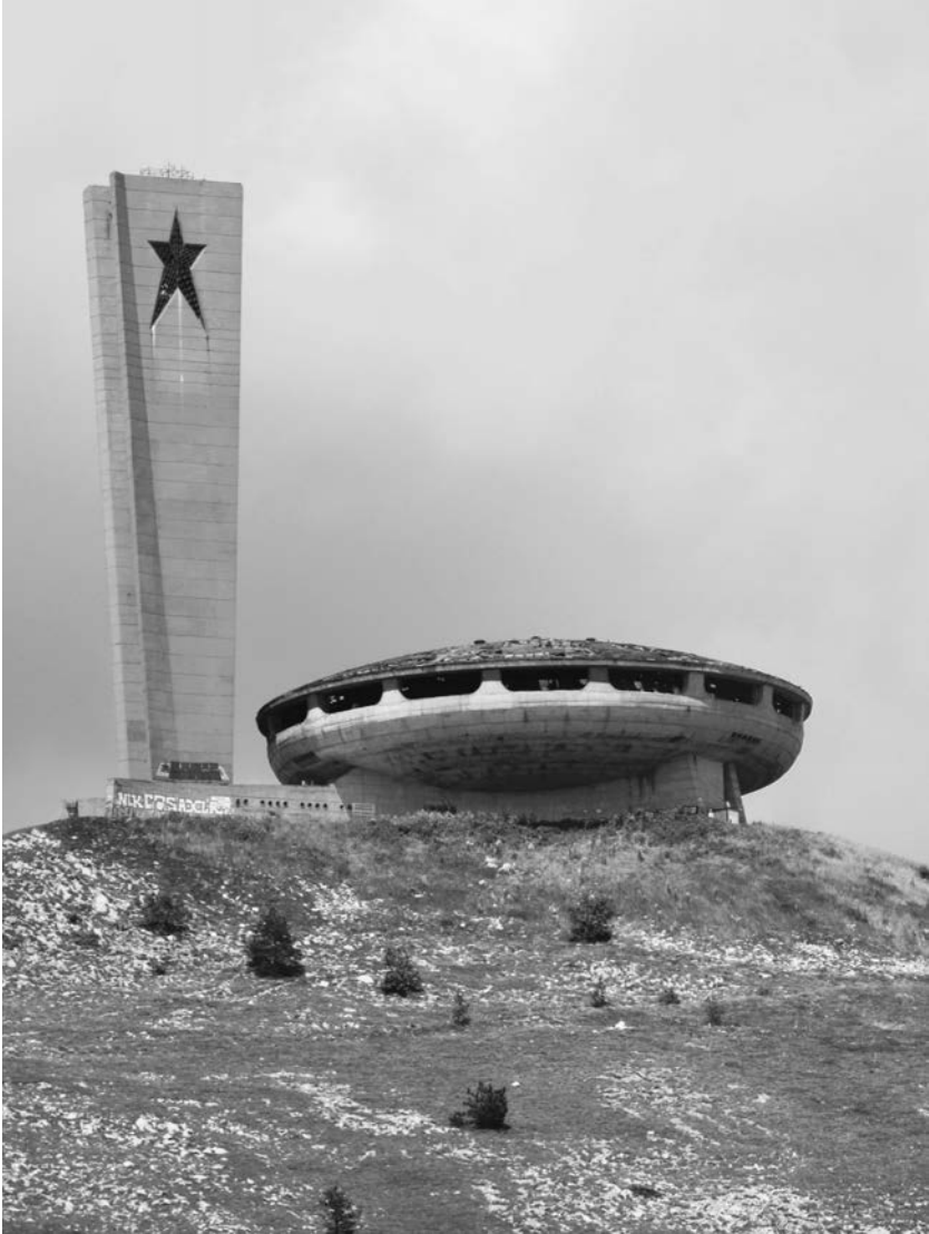
FIGURE 40. The Home Monument of the Party on Buzludzha in summer 2019. The graffiti, damaged ceiling, and missing red star are visible even from a distance. Photo by author.
