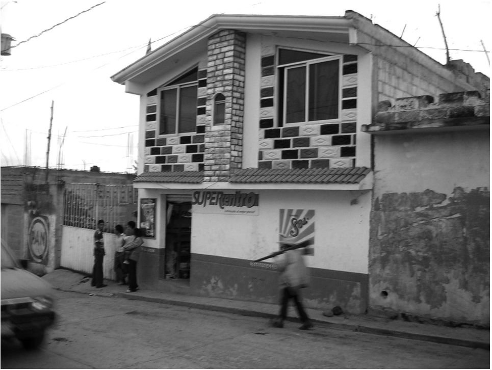
FIGURE 5.2. A “remittance house,” shop, and bakery built by early migrant Efen Tellez’s family in San Mateo Ozolco, Mexico. (Photo by Domenic Vitiello, 2007.)
