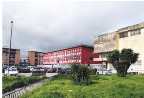
FIGURE 8 (LEFT) CEP-Traiano, view of the square of the “social-trade centre” by Marcello Canino, 2019
