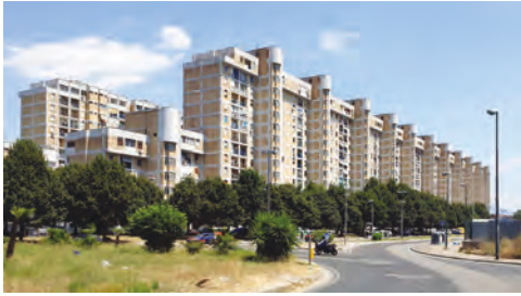
FIGURE 7 Scampia. Housing complex north of “Le Vele,” 1980. Photo 2019 (ed.)
