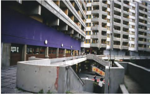
FIGURE 14 Terraced basement of Kottbusser Tor square in NKZ, 1987 (ed.)
