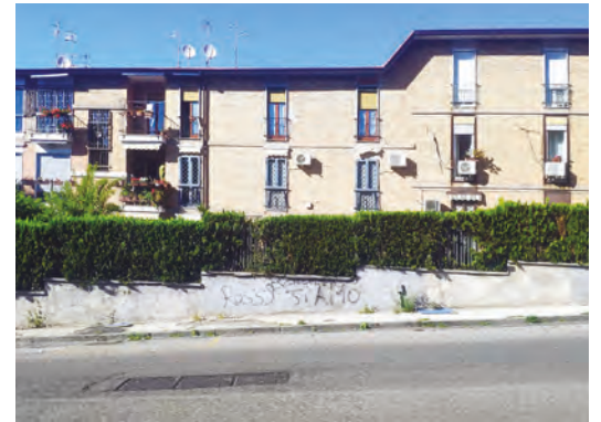
FIGURE 13 North sector, Via Adige, 2020
