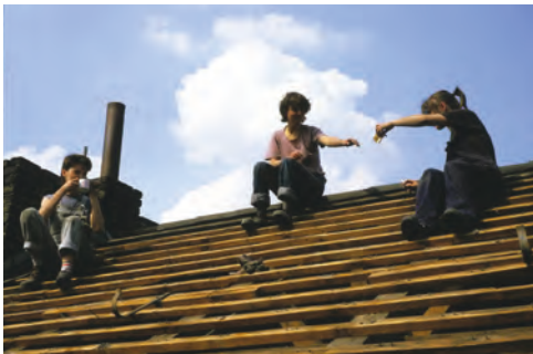
FIGURE 6 IBA-Altbau, self-construction site on the roof of “Schokofabrik,” 1985 (ed.)
