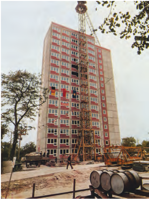
FIGURE 19 Cherkassy, Ukraine. Type "Erfurt" under construction. Photo by Thomas Billhardt, 1978
