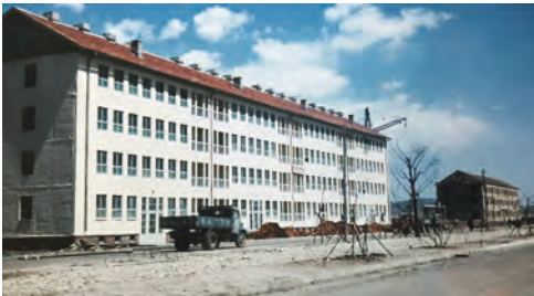
FIGURE 7 (ALL ABOVE) Hamhung. Gallery house (above), house built with jumbo blocks (centre), house built with concrete panels (below), ca. 1950
