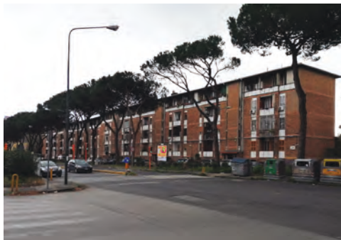
FIGURE 11 CEP-Traiano, typologies of housing: four and five-storey buildings on Viale Traiano. Photo 2019
