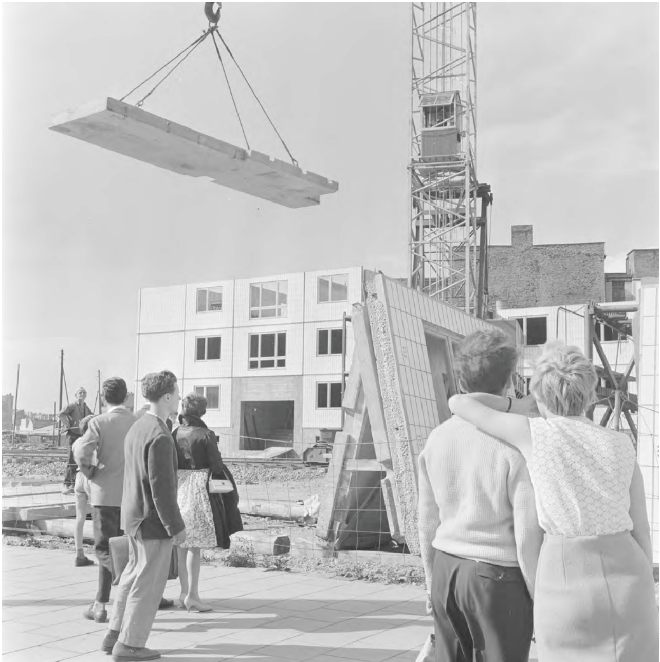
Building site of Karl-Marx-Allee near Alexanderplatz. Photo by Horst Sturm, 1960
