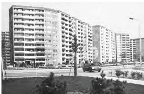
FIGURE 9 Housing buildings along Mehrower Allee. Photo by Monika Uelze, ca. 1982
