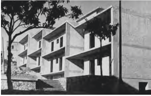
FIGURE 5 Type 10 under construction, 1949–51
