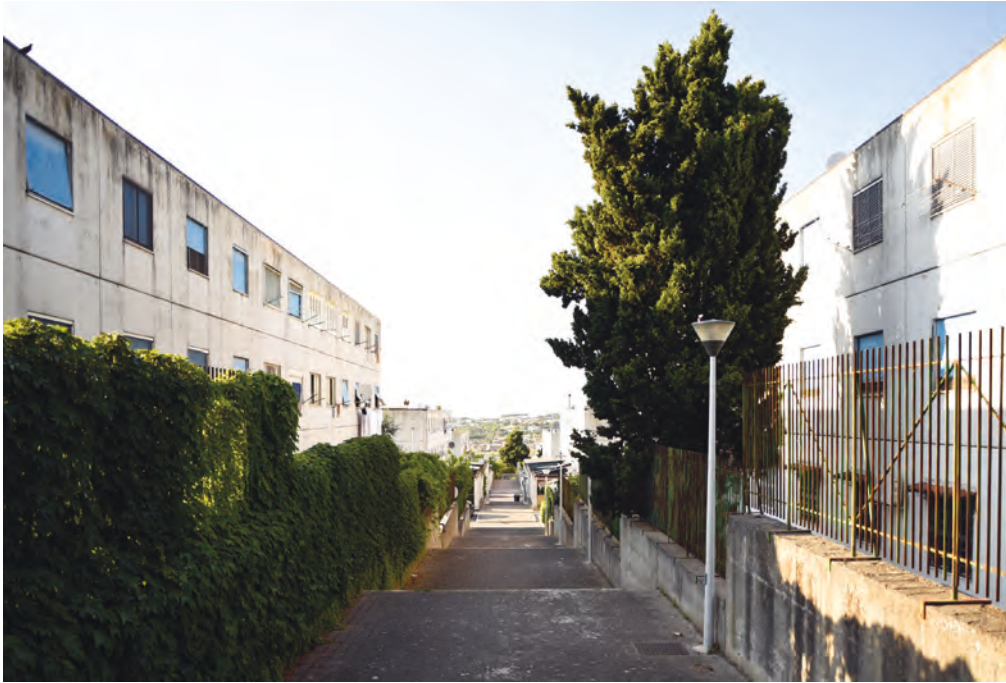
FIGURE 11 (LEFT) Connecting pathways and housing units, 2019
