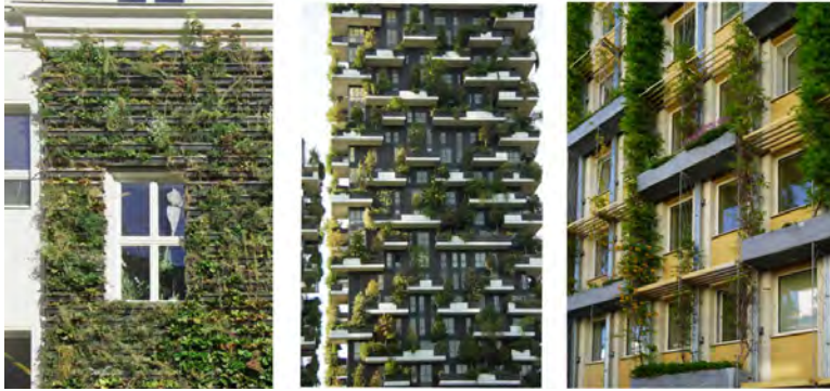
Figure III.2: Pot-based green facade directly attached to the facade (left) on balcony (middle) and on supporting structure with climbing aid (right) (images by Irene Zluwa)
