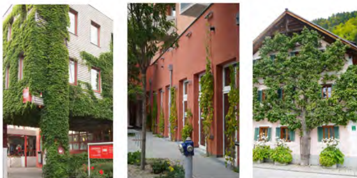
Figure III.1: Ground-based green facades with self-clinging climber (left), on climbing aid (middle), and trellie-tree (espalier tree, right) (images by Irene Zluwa)
