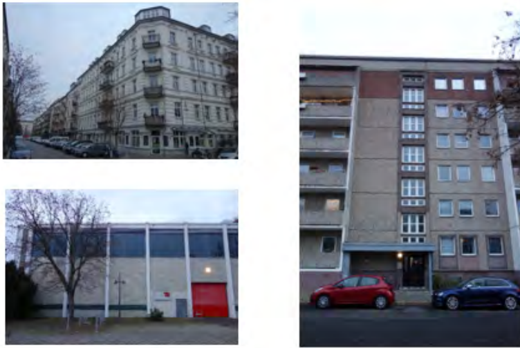
Figure IV.23: top left: Wilhelmine building, Prenzlauer Berg, Berlin, Germany; bottom left: test hall at TU campus, Berlin, Germany; right: pre-fabricated panel building, Berlin, Germany (images by Karin A. Hoffmann)
