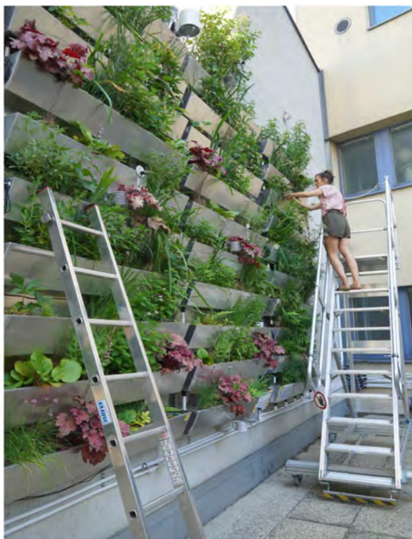
Figure IV.5: Staircase for the accessibility of the VGS at the University of Natural Resources and Life Sciences, Vienna (BOKU) (image by Irene Zluwa)
