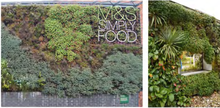
Figure III.3: Modular (left) and continuous (right) wall-based green facade (images by Irene Zluwa)
