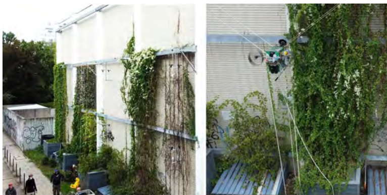
Figure III.20: Test site before (left) and after (right) the first cut (images by Sebastian Schröder)
