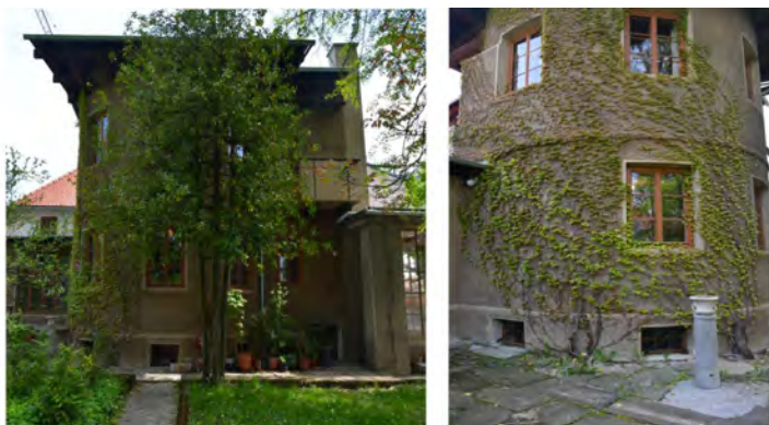
Figure V.11: Plečnik house in Ljubljana, where greened wall ( Parthenocissus tricuspidata ) as a part of original design was preserved after renovation in 2015 (image by Damjana Gantar)
