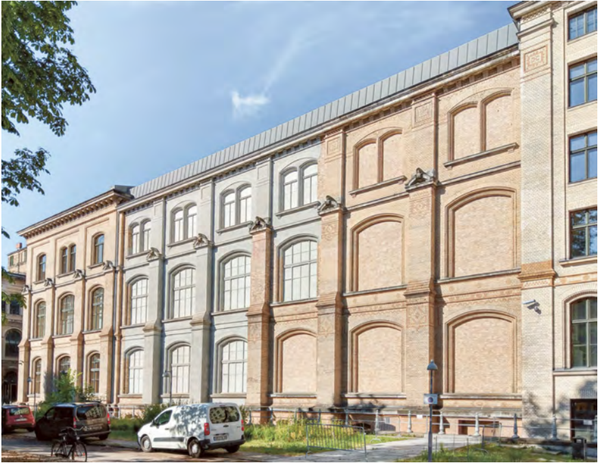
Fig. 8: Natural History Museum Berlin – reintegration of the missing gap by mimetic repetition of the original structure in visible cast concrete, Diener & Diener Architekten, photo 2021.
