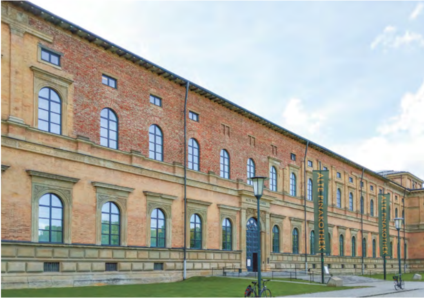
Fig. 4: Alte Pinakothek Munich – Hans Döllgast’s reintegrated north façade with bare re-used bricks and lack of decorative elements, photo 2021.
