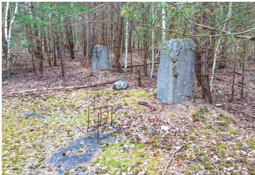
Fig. 4: Concrete floor at Fertigungshalle 1 (F1) (6 September 2021).
