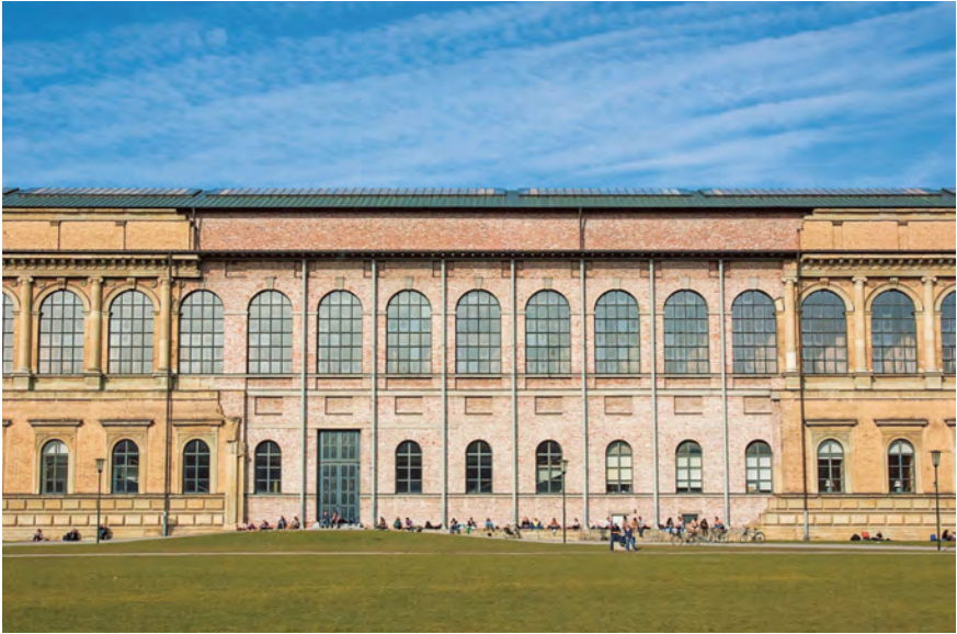
Fig. 3: Hans Döllgast, Alte Pinakothek (reconstruction), Munich, 1946–73, recent photo.
