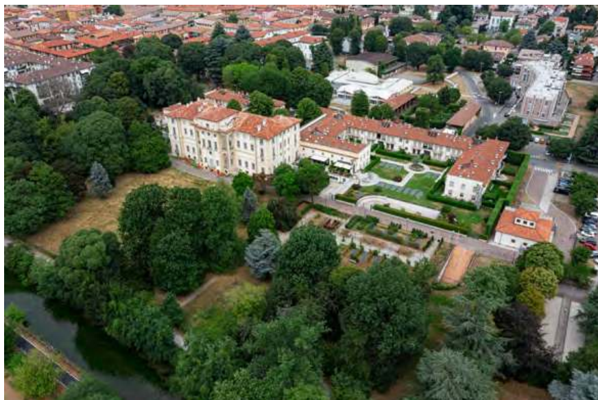
Fig. 5. Villa Alari Visconti (Cernusco sul Naviglio) (courtesy of Imerio Raffaini, reproduced with permission).
