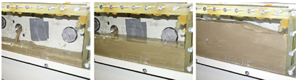
Fig. 5.46 Filling of the annular gap with a two-component grout commonly used in practice (reference grout M0, activator content: 90 kg/m 3 , gel time: approx. 9 sec.) [69]
