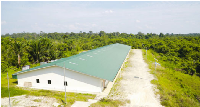
Fig. 15.14 The current Melilas longhouse, built under the Julangan Titah project funded by the Sultan of Brunei. Source Personal collection of Azlin
