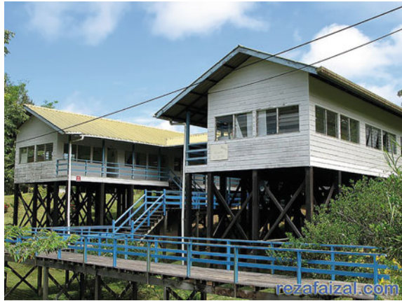
Fig. 15.3 Melilas Primary School, built on stilts to avoid flooding. Source Personal collection of Azlin
