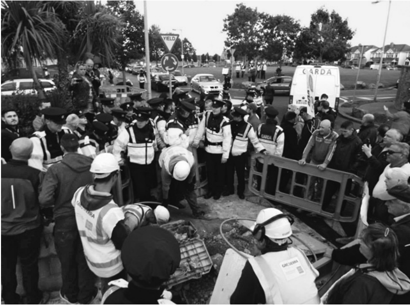
2.1 Water meter installation in Dublin, 2014. (Image courtesy of Dublin Says No.)
