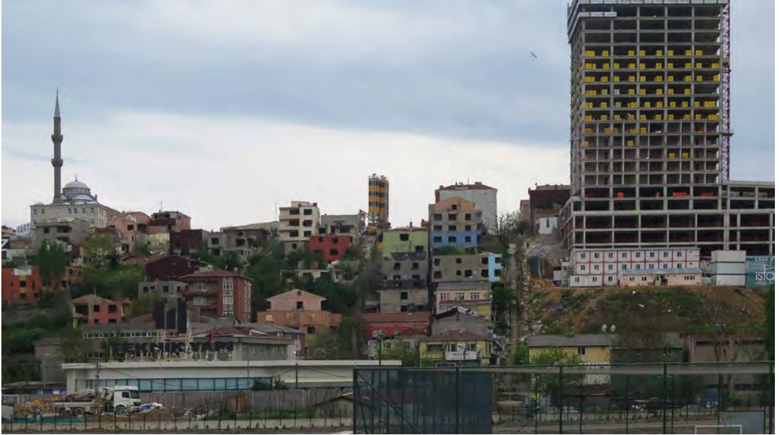
➊ Fig. 4 An emptied-out neighborhood, slated for demolition, stands beside a construction site in early 2017. Mosques and some schools are the only buildings spared from demolition in redevelopment areas—and not always (photo: Francesco Pasta, Fikirtepe, Istanbul, April 2017).
