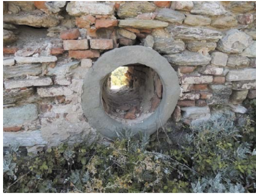
Figure 6 – A fire mouth realized in Pietra Serena sandstone.
