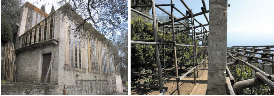
Figure 4 – A limonaia in Gargnano, recently restored following historic construction techniques and using past materials and maintained according to traditional methods, then closed and covered in the winter months.
