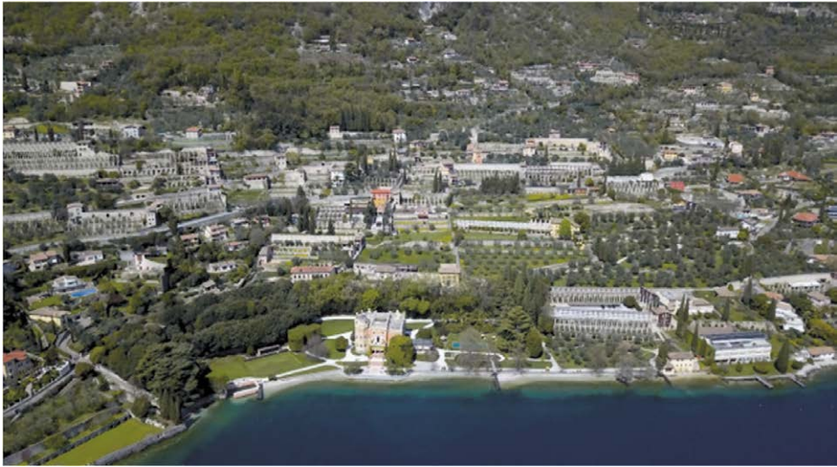
Figure 3 – Gargnano (Brescia, I) today: this photo shows how much the limonaie (clearly recognizable by the terraces and pillars) still characterize the upper Garda landscape.
