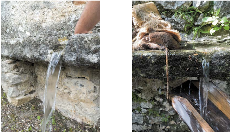
Figure 7 – Two activated spillways at the limonaie Ragusini (left) and Fondo Crocefisso (right).
