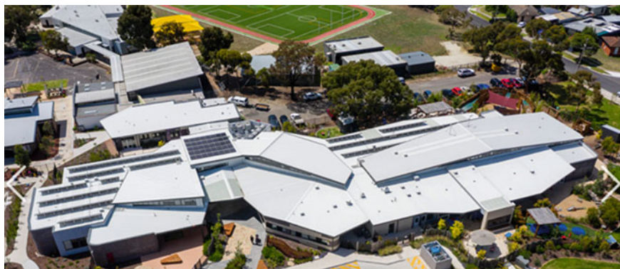
Fig. 1 Aerial view of Korayn Birraleee Family Centre, with connection to Northern Bay P-12 College (Image courtesy of Brand Architects. Photograph by Blue Tree Studios)
