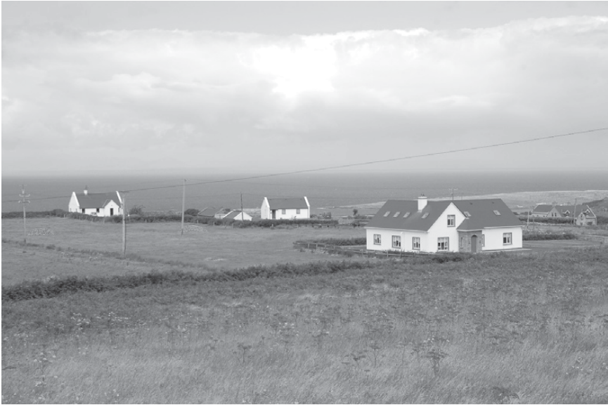
Figure 7.1 Dispersed rural housing in County Clare, west of Ireland.
