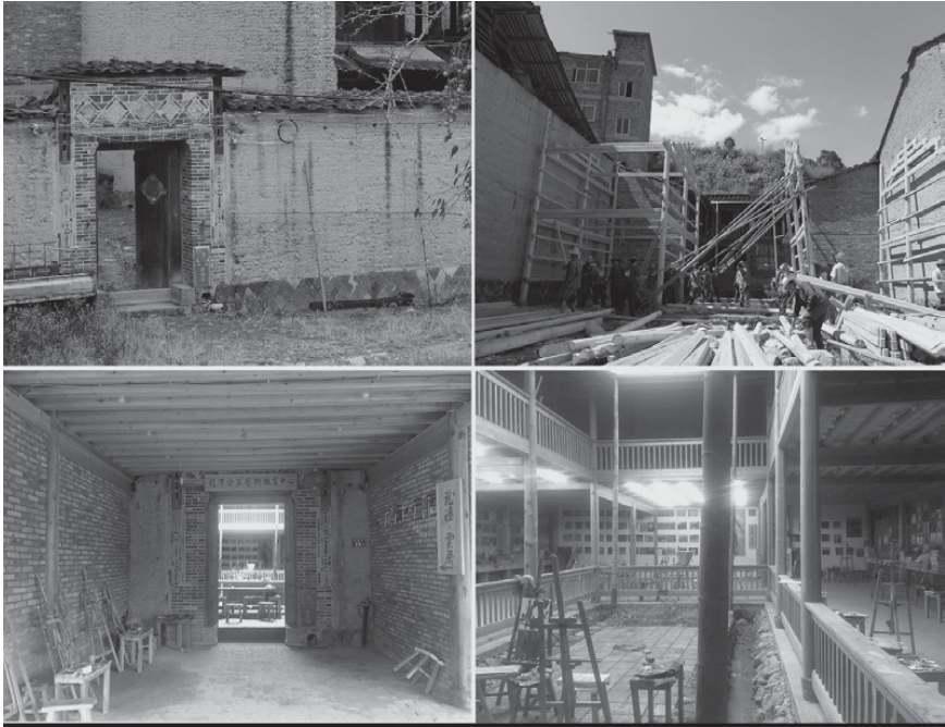
Figure 10.2 Longtan Public Art Education Center before, during and after renovation, 2017.
