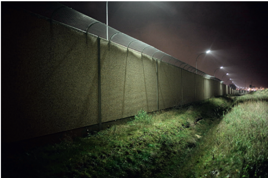
Figure 8.5 Calais, France, June 2017. The Great Wall of Calais: a four-meter high and one-mile long anti-intrusion barrier surrounding the Calais port. The British government funded the construction of this wall. Photo: Eric Leleu.
