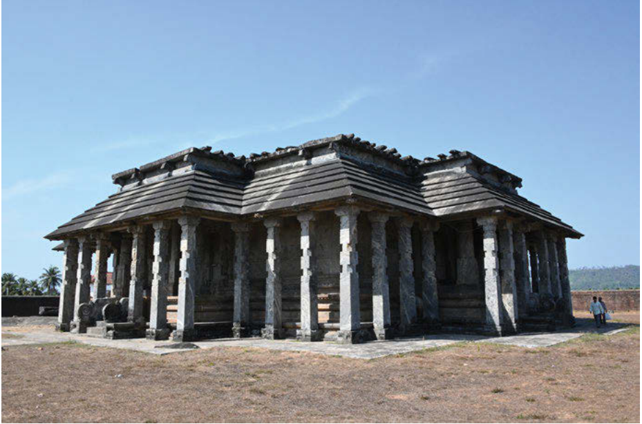
Plate 3.6: The heavy stone roof of the Caturmukha Basti at Karkal is supported by a large number of stone pillars from below.
