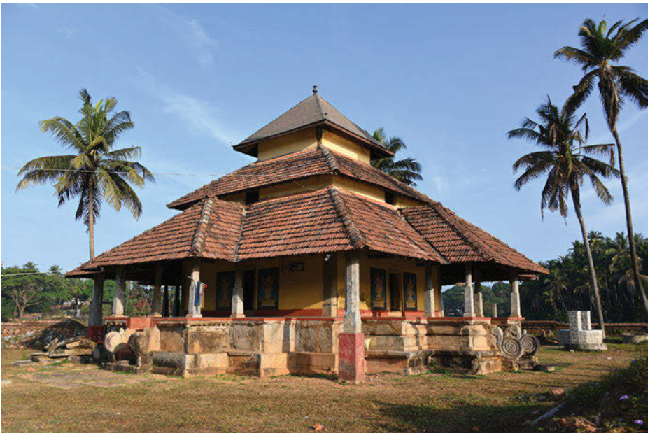
Plate 3.4: View of the Kere Basti near Karkal, which has multiple sloping roofs protecting the wood and mud-built construction against the rains.
