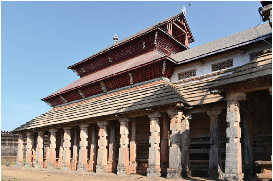
Plate 3.8: At Mudabidri, the two-storeyed Guru Basti and the triple-storeyed Candranātha Basti show combinations of stone and wooden floor levels.
