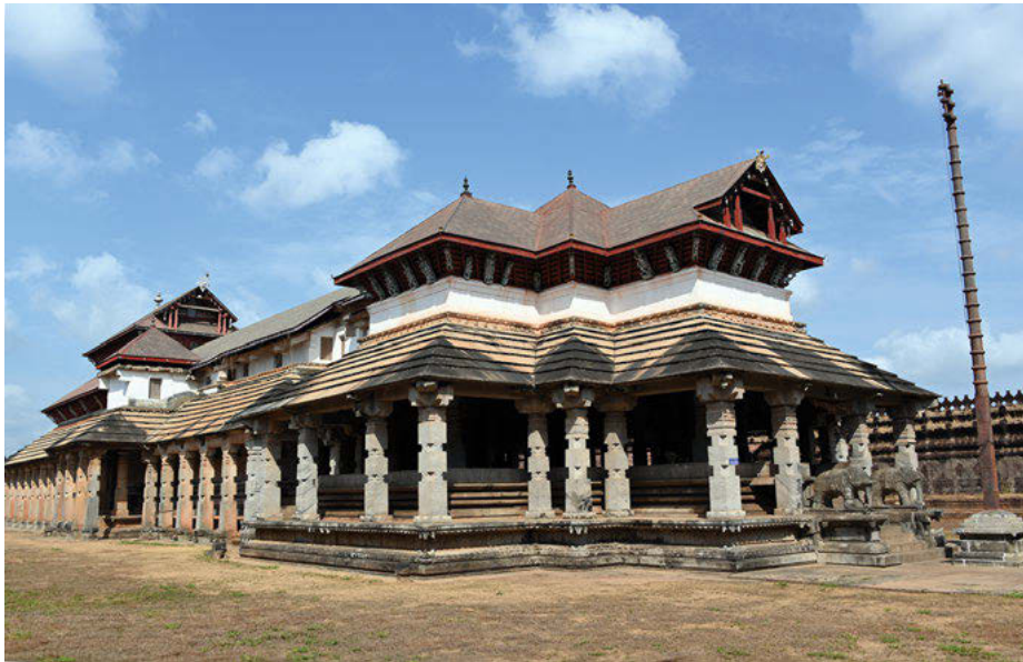
Plate 1.3: Mudabidri, coastal Karnataka. Reflecting a strong dependency on the climate of strong monsoon rains, the temples have multiple slanting and projecting roofs.
