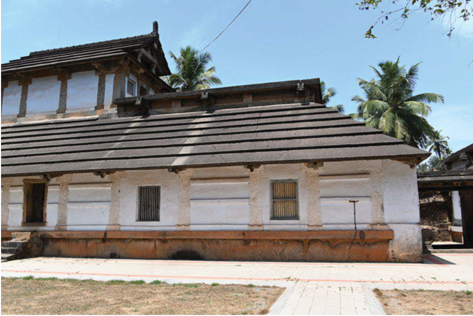
Plate 3.9: The Baḍaga Basti at Mudabidri is almost entirely made of stone, including its raised storey.
