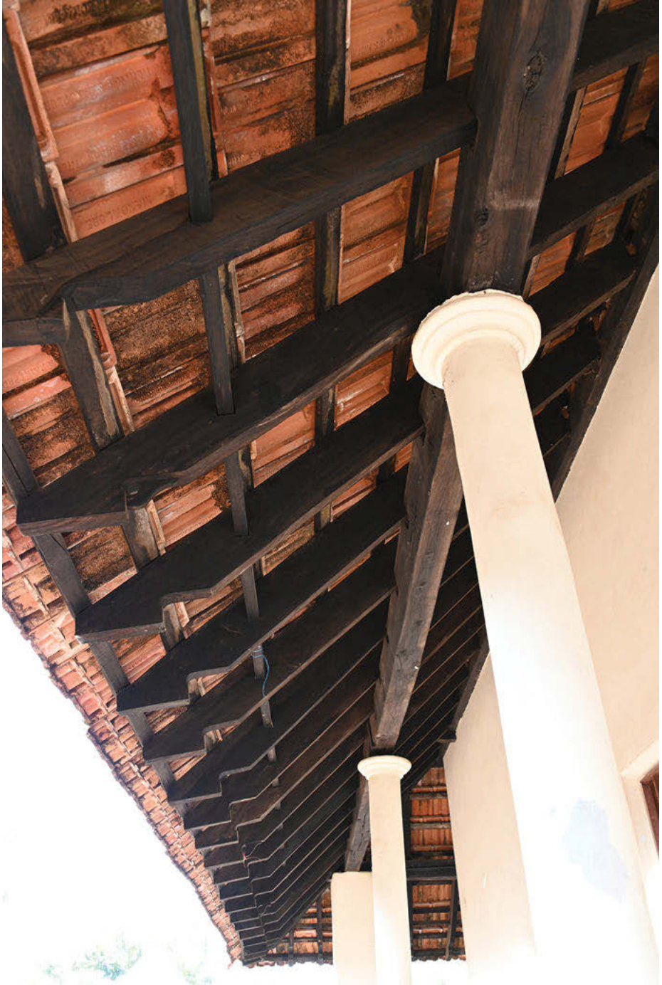
Plate 3.5: View into the roof of the Pārśvanātha Basti at Venur, revealing its wood and tile construction.
