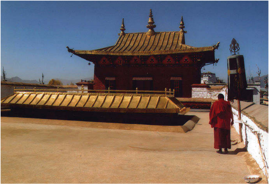
Plate 11.3: Ramoche roof terrace upon completion of waterproofing of terrace, 2006.
