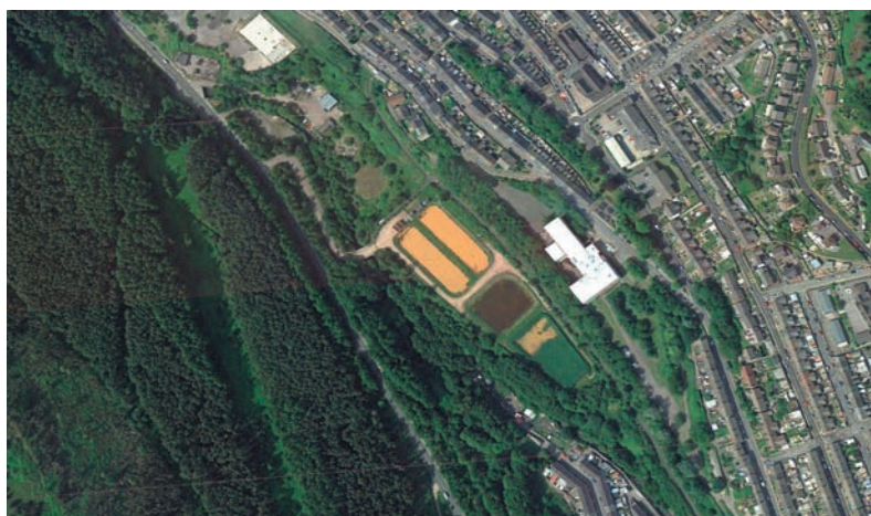
Figure G.1 Six Bells Mine Water Treatment Scheme 51°43 33.56 N 3°07 58.63 W 638 m. ©2019 Google.
