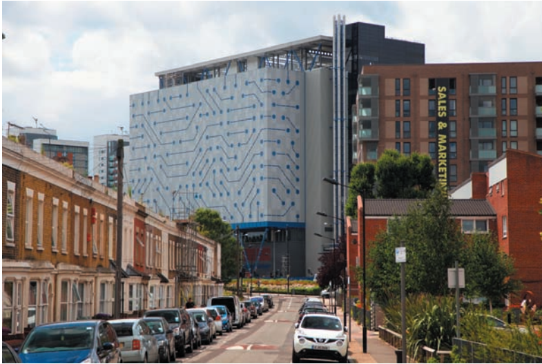
Figure D.1 Tom Ravenscroft, TeleHouse North 2 at East India Dock campus , 2016. Courtesy of the architect.
