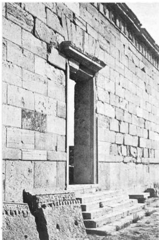
(a) Forum: entrance from the street at the north corner. Note the orthostate course at the base of the wall and the ornamental drafting of the masonry above.
