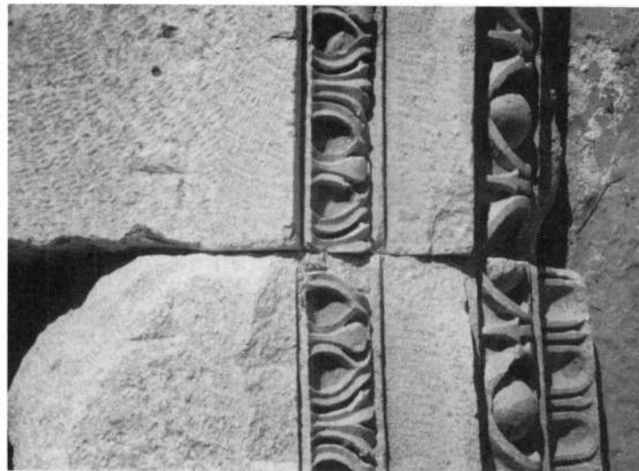
(c) Assembly marks on cornice of basilica apse.
