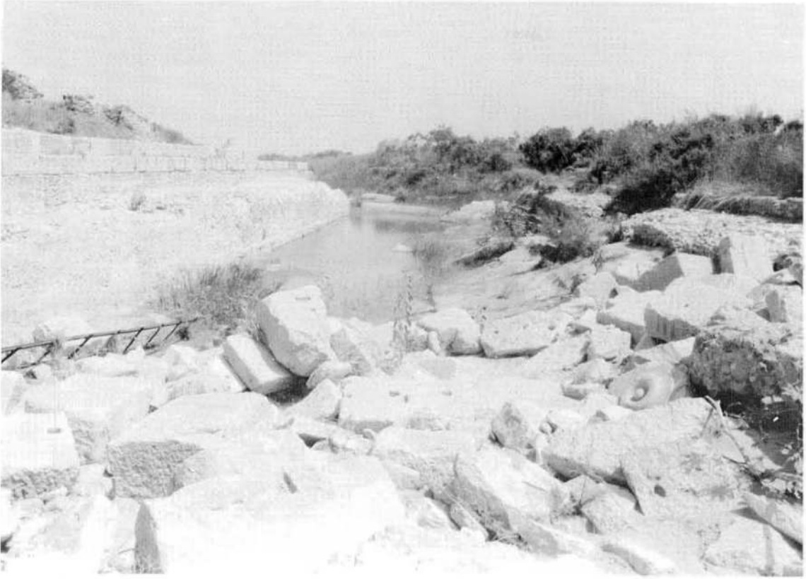
(a) The Colonnaded Street: looking inland after the flood of 6 November 1987.
