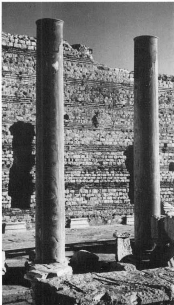
(a) Forum: rear wall of the tabernae on the south-east side, showing the surviving pilaster bases of the veneer decoration and entrances cut through the wall in the Byzantine period.
