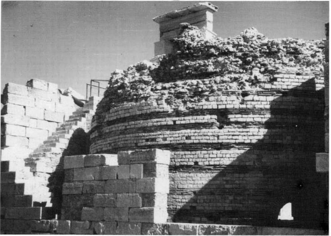
(a) Basilica: north-west apse from behind.
