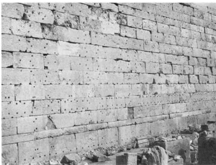
(d) Forum: fixing-holes for the veneer on the inner face of the north-west perimeter wall.
