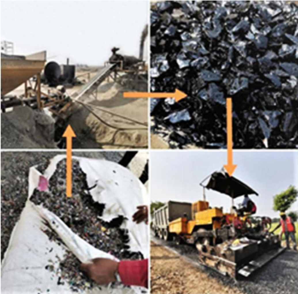
Figure 6.58 Incorporating PW into a road asphalt mixture using the dry process (Source: Heriawan, 2020).
