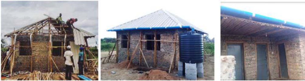
Figure 6.55 Demonstration of Bottle House Project, Nigeria (Source: Oyinlola et al., 2018 ).
