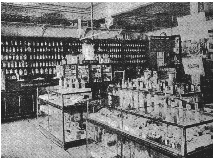
Figure 1.5 Interior of Thomson & Taylor, Chemist and Druggist , Bombay
