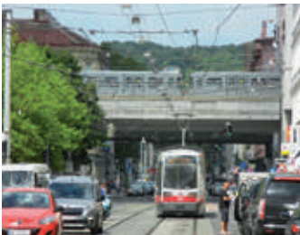
The view of the Gallitzinberg Hill from the depths of Thaliastrasse would have been largely lost if the turnaround facility had been enclosed.
