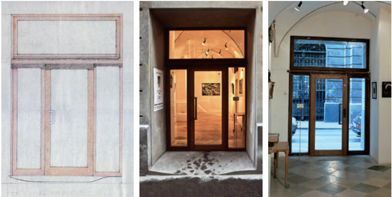
The passive leaf, the active leaf and the fixed part of the portal (from left to right) are not standardized, but set apart from one another.
