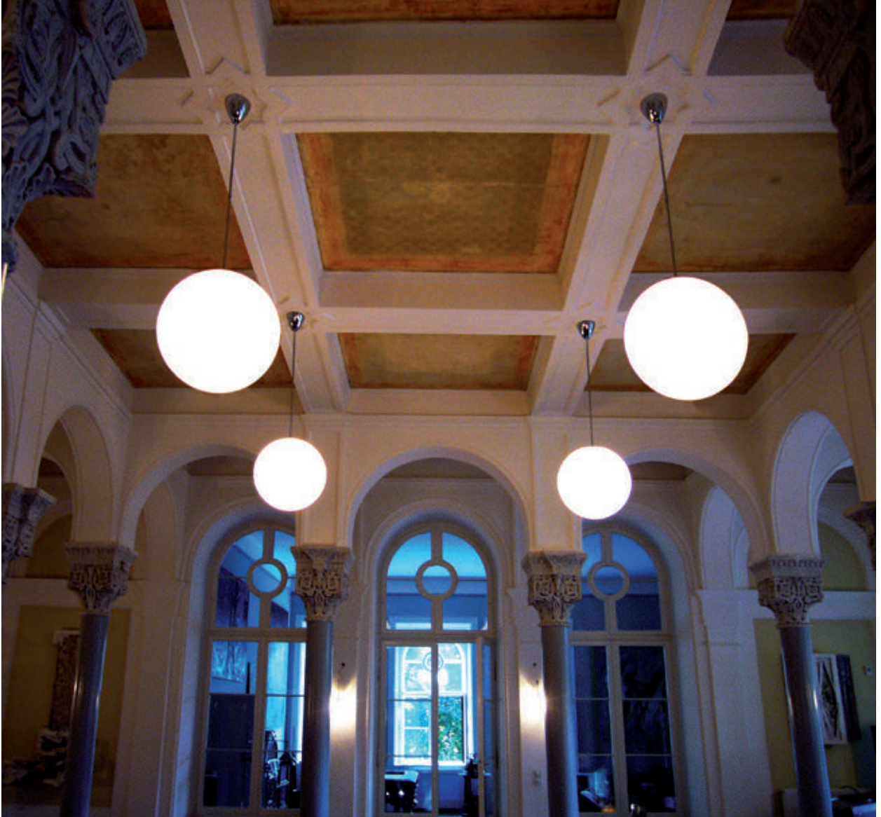
The basis of the restoration was the rudimentarily preserved painting of several ceiling fields.
