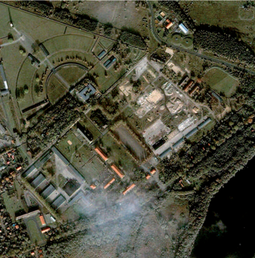
The site after ca. 2002: The buildings erected after 1945 were demolished, thereby removing the traces of subsequent use by the NKVD (Soviet Secret Service) and NVA (GDR Army).
