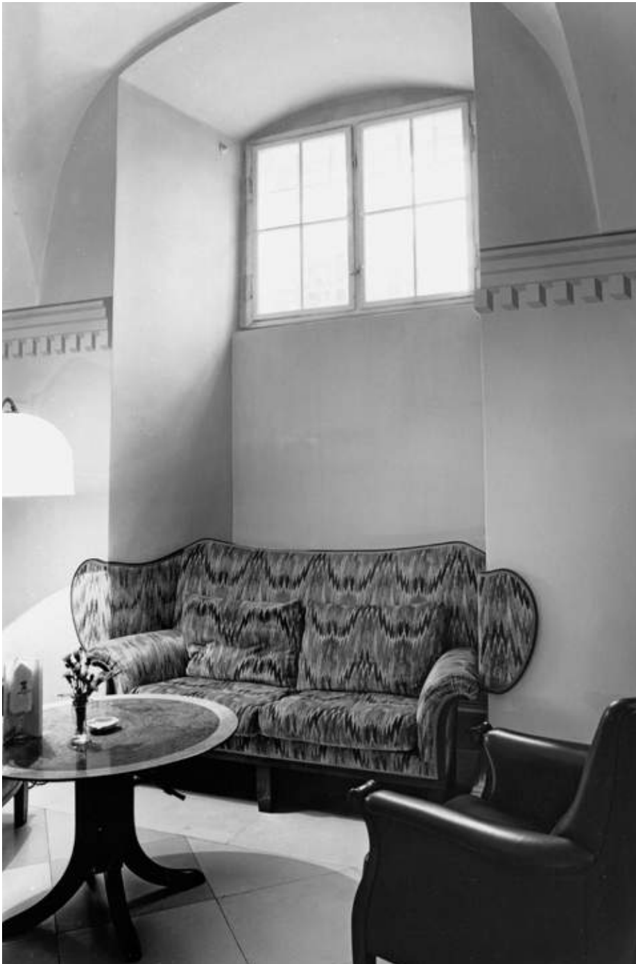
The cornice on the wall is painted; only the perspective projection of a "tooth" on the corner of the wall is actually implemented.
