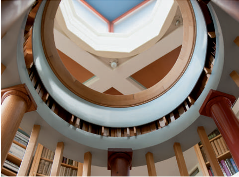
The book edges in the parapet create the dentil of the cornice profile.
