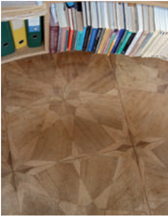
Parquet boards from a demolition with a diagonal and half-diagonal pattern
