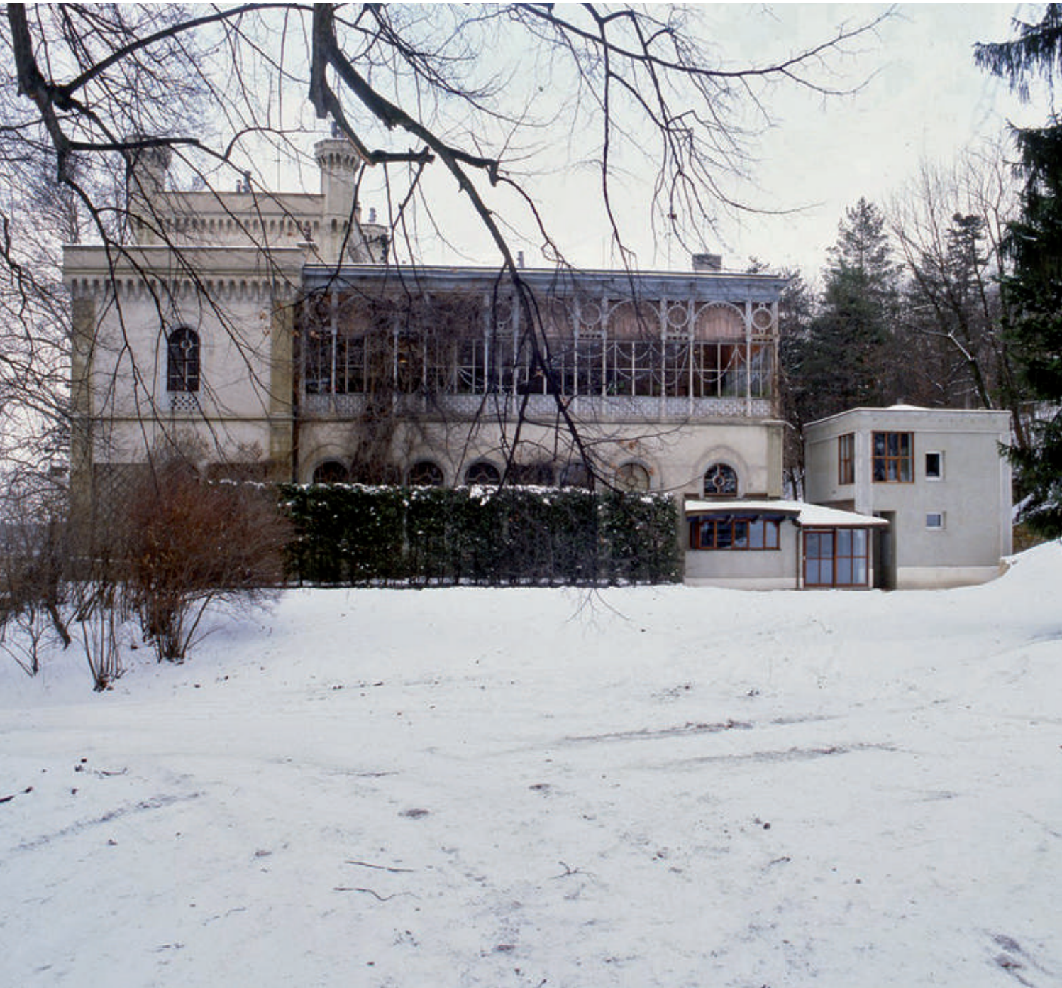
The structure of the new southern front now corresponds to that of the original northern front.
