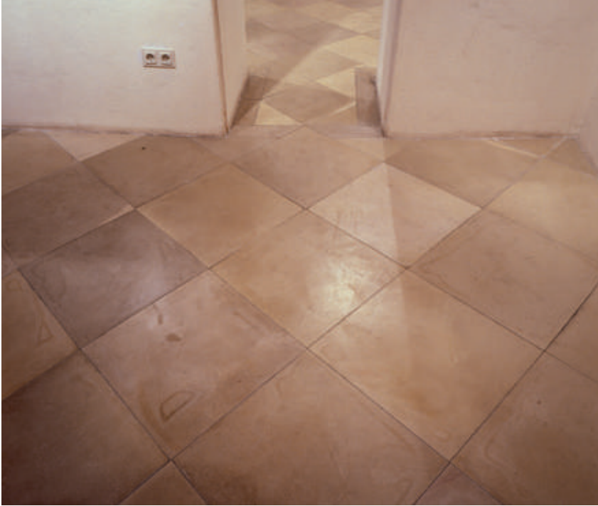
Various panel formats and edging differentiate the two rooms as older and younger, but also as more intimate and formal.
