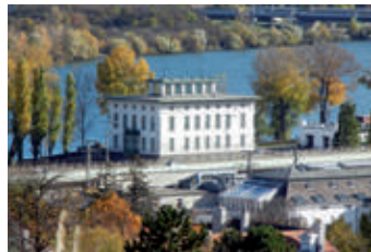
Otto Wagner: Administration building for the Nussdorf weir and lock system, 1899 – the roof attachment served as an observation station.
