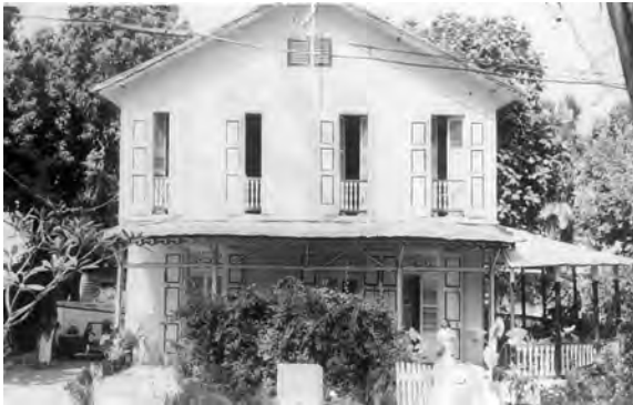
My grandparents' gingerbread home on Rue Duncombe in the Bois Verna neighborhood, damaged and later demolished following the 2010 earthquake. (AC d'Adesky)
