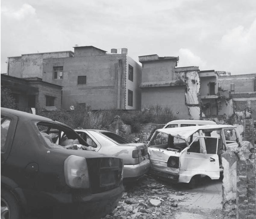
FIGURE 21. Partially demolished housing and cars damaged by a demolition bureau. Photo by author.
