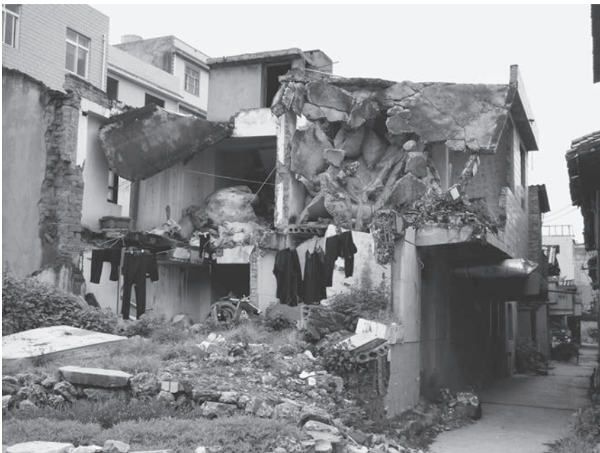
FIGURE 20. A partially demolished house. Photo by author.
