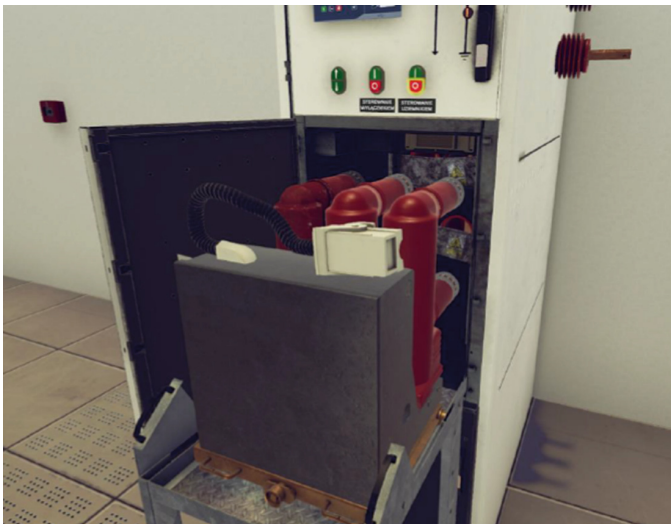
Fig. 6. The MV circuit breaker in VR application
