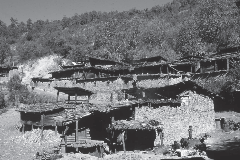
FIG. 3.1. Cluster of houses in Bustling Township. The roofs are made of planks kept in place with stones. While these houses are made partially of stone, in many areas of Bustling Township, houses are made entirely of logs.
