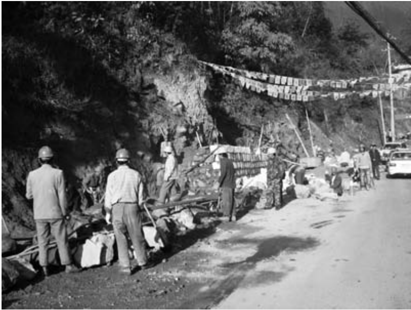
FIG. 4.3. A team of migrant workers from Dali Prefecture constructs retaining walls along the main street of the Gongshan county town (December 2006).
