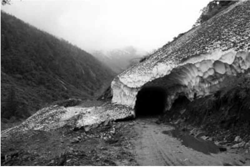
FIG. 1.2. The road connecting Dulongjiang township with the county town. Even in summer, some sections remain covered in snow and ice (July 2005).
