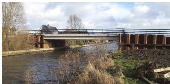
Figure 2. Temporary access bridge Oling 5: reused girders, sheet piles and purlins.
