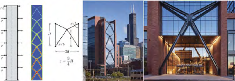
Figure 22. Lateral frame concept and final construction of 800 West Fulton Market, Chicago.
