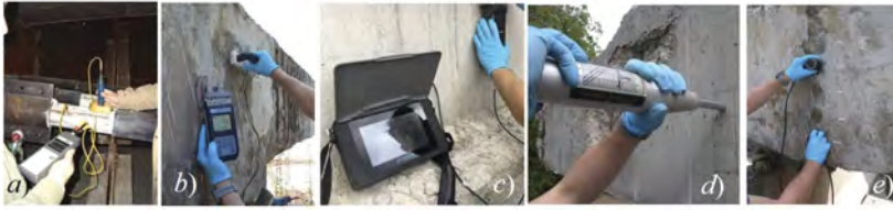
Figure 6. Examples of non-destructive tests: (a, b), electrochemical inspection techniques; (c) concrete cover measurement; (d, e) Schmidt rebound hammer and ultrasonic pulse tests.
