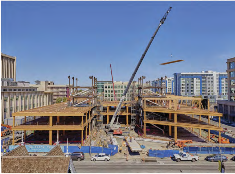
Figure 8. COB3 Construction showing steel frames in mass timber construction.
