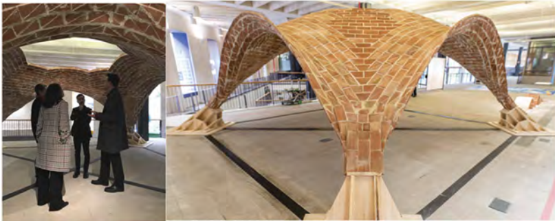
Figure 12. Constructed masonry timber vault indicating material removal and overall geometry.
