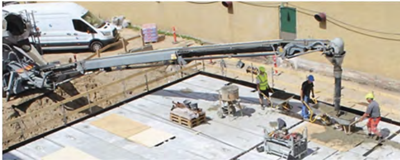
Figure 1. Ordinary pouring of joints in a precast concrete building.
