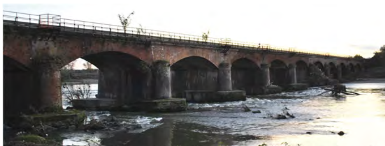
Figure 1. The Candia bridge: view from the upstream of Sesia River.
