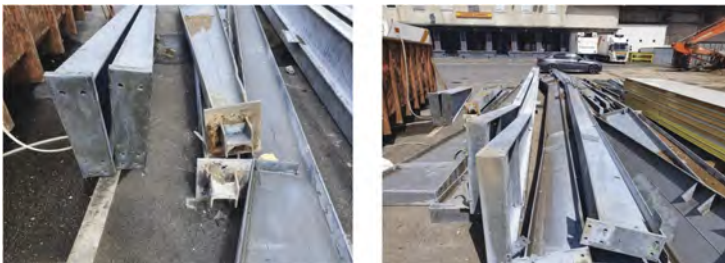
Figure 12. Deconstructed parts of primary structure ready to be reused.
