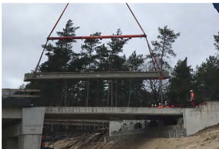
Figure 3. Placing the reused girders in Hoog Burel.
