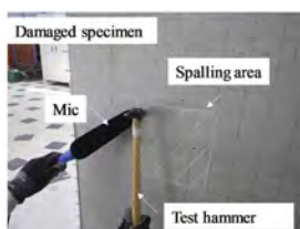
Figure 1. Example of a hammering test at spalling concrete in a damaged specimen.
