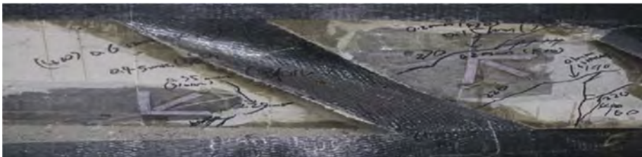
Figure 4. Experimental phenomena of concrete beams strengthened with obliquely bonded carbon fiber strips.
