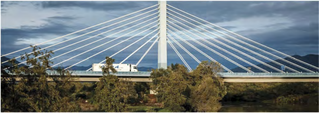
Figure 1. Overview of cable-stayed bridge over Garigliano river.
