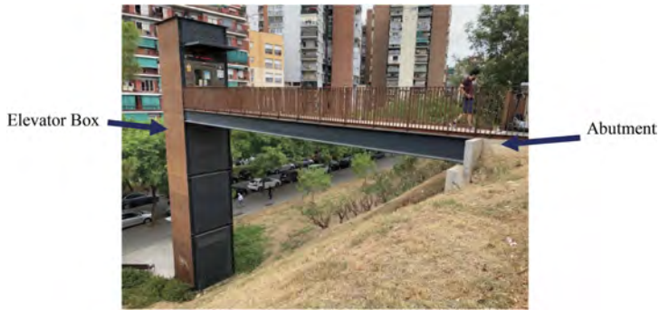
Figure 3. A picture of the pass way bridge.
