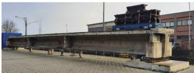
Figure 1. The prestressed bridge beam under study.
