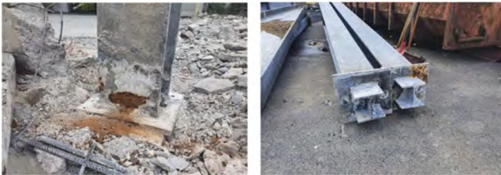
Figure 11. Removing concrete at jointing of steel arcs.
