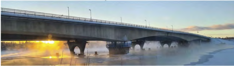
Figure 1. The old Kalix bridge in the foreground with foundations of the new bridge behind.
