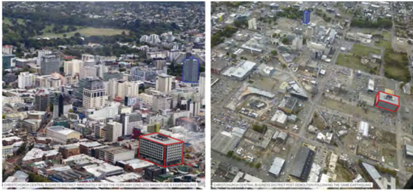
Figure 1. Damage and demolition of buildings - Christchurch, New Zealand due to the 2011 earthquake.
