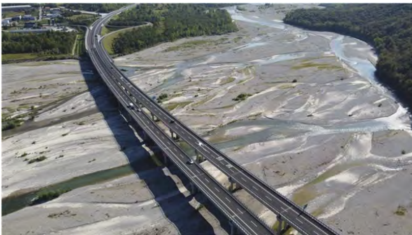
Figure 2. An example of geotechnical asset difficult to reach, in this case the inspection concerns the slope below the highway, that in this particular case is the riverbed.
