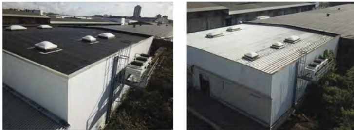
Figure 8. Removal of roof insulation and sealing; Left picture before removal.
