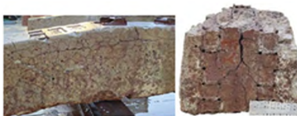
Figure 2. Crack pattern in the shoulder of a prestressed concrete sleeper.
