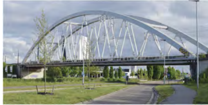
Figure 1. The KW51 bridge, as seen from its north side.
