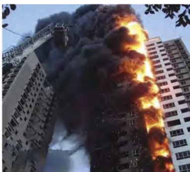
Figure 2. Fire incident caused by the insulation layer.
