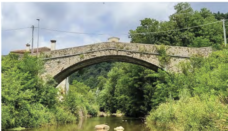
Figure 1. View of the bridge.
