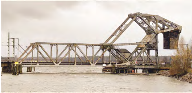
Figure 1. A photo of the Vänernsberg Bridge.
