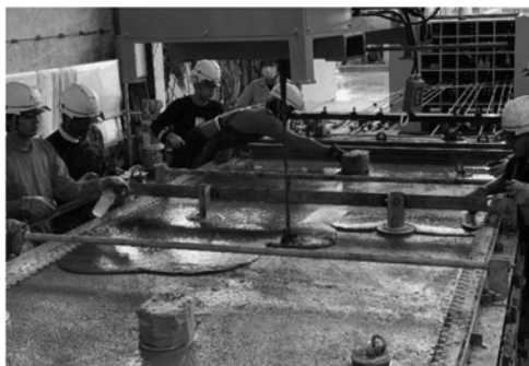
Figure 14. Powering of UFC on fresh concrete.
