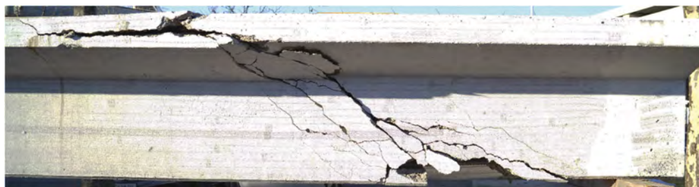
Figure 8. Photograph of fatigue failure of tested beam.
