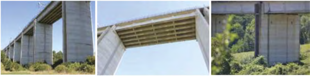
Figure 1. High-speed railway bridges with PC grillage decks and RC piers.
