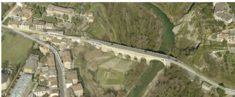
Figure 1. Aerial view of the SS Filippo and Giacomo bridge.
