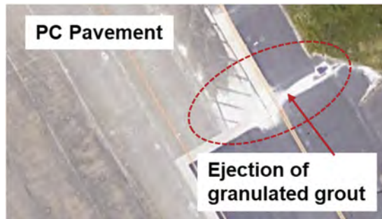
Figure 1. Ejection of granulated grout at airport PC pavement.
