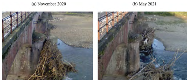
Figure 5. Pictures from the permanently installed cameras: (a) debris accumulation on P05 in November 2020 resulting from the important event of October 2020; (b) debris accumulation on P05 and P04 after the event of May 2021.
