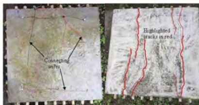
Figure 2. Slab protected by galvanic anodes (left) and corroded slab without anode protection (right) showing extent of cracking of the concrete caused by steel corrosion after exposure to outdoor warm and humid conditions for over 10 years.
