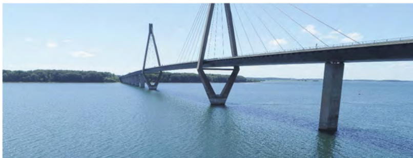
Figure 5. The Faroe Bridges (Cable Stayed Bridge in South).
