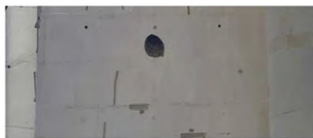
Figure 7. Panoramic splicing of beam bottom.
