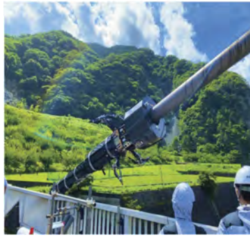
Figure 7. On-site verification of the cable inspection robot.
