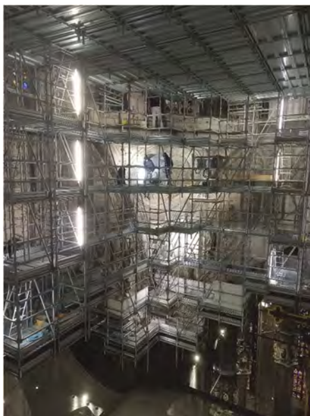
Figure 1. The scaffolding for the Tiburio restoration.
