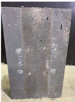
Figure 4. Failure mode of S-16-150-h90 specimen.
