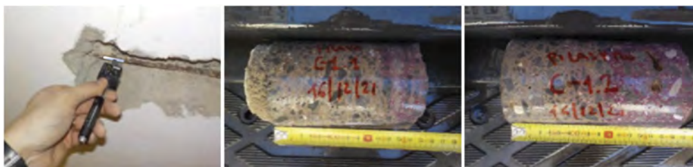
Figure 4. Leeb rebound hardness test and concrete samples.
