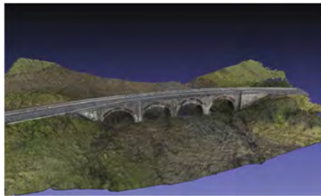
Figure 3. 3D point cloud of the Maletto Bridge.
