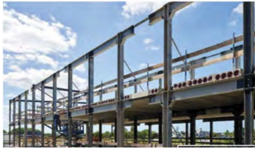
Figure 3. Construction of Biopartner 5, whereby steel elements are used from the neighboring Gorlaeus-building (Terwel et al. 2021).
