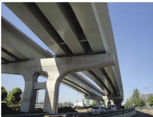
Figure 1. The typical OSD bridge selected for investigation (courtesy of Dr Junlin HENG).
