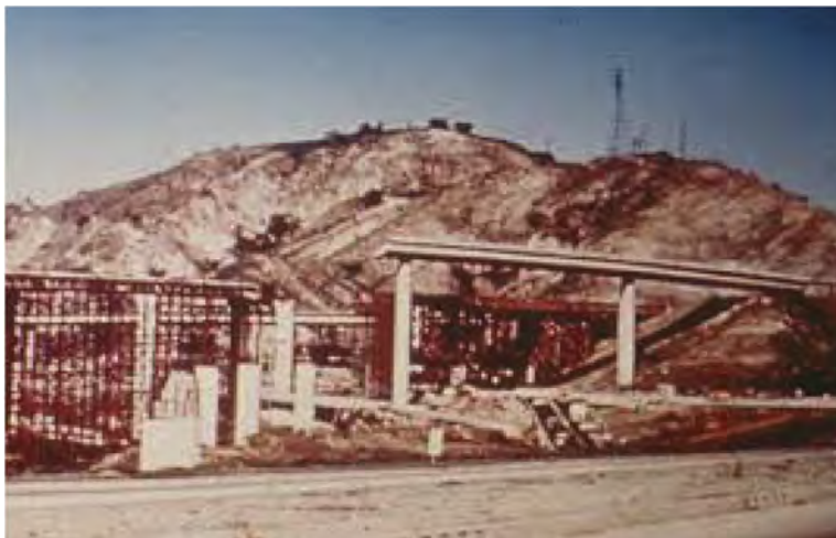
Figure 2. The collapsed sections of South Connector Overpassing after the San Fernando Earthquake (Shirazi 2015).
