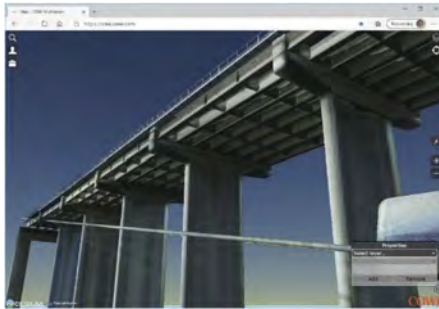
Figure 2. Reality capture of approach spans at the New Little Belt Bridge.
