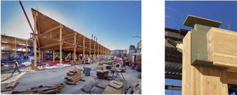
Figure 18. COB3 project under construction and typical beam-to-column connection detail.
