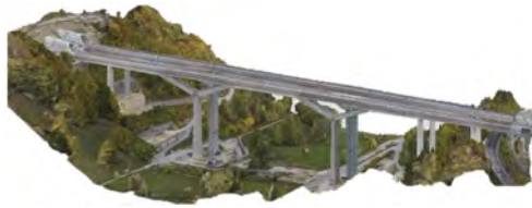
Figure 1. 3D scan of the right Filstal bridge.
