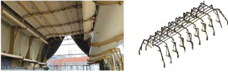
Figure 2. Café Horta, interior view (left), captured point cloud after steel segmentation (right).
