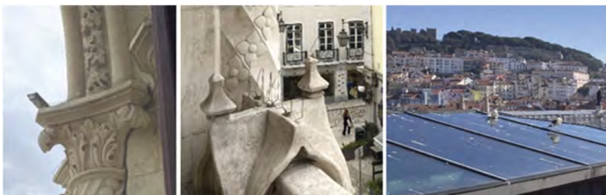
Figure 2. Existing bird deterrent system (a, b); skylight with permanence of seagulls (c).
