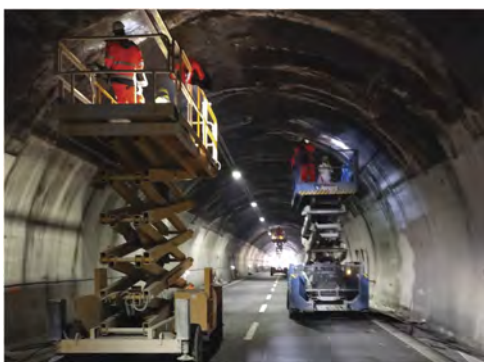
Figure 1. Inspection of the tunnel lining with MEWP.
