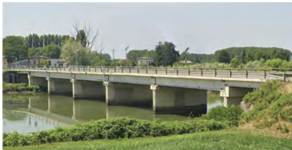
Figure 1. The Isola Dovarese bridge.
