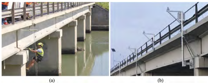
Figure 6. (a) Installation phase (b) GeoGuard Monitoring Units and steel supports.
