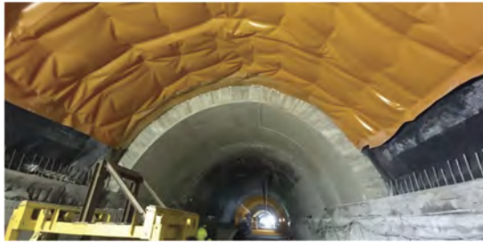
Figure 5. Examples of lining reconstruction.
