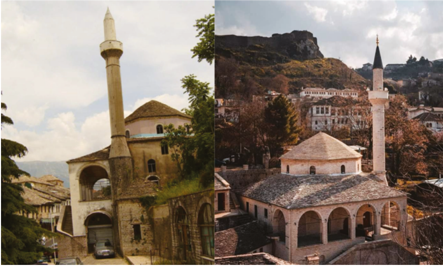
FIGURE 6.27 Image of Mosque of Bazar in Gjirokastra in 2005 (left) and after restoration 2021 (right)
