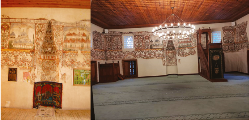
FIGURE 6.22 Mihrab image in 2005 (left) and after restoration qibla inner façade in 2021 (right-KMSH)
