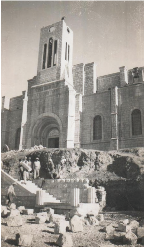
Fig. 6.2 The construction of St. Mary's Church in Kfarsghab, 1948. (Photo provided by James Haddad)
