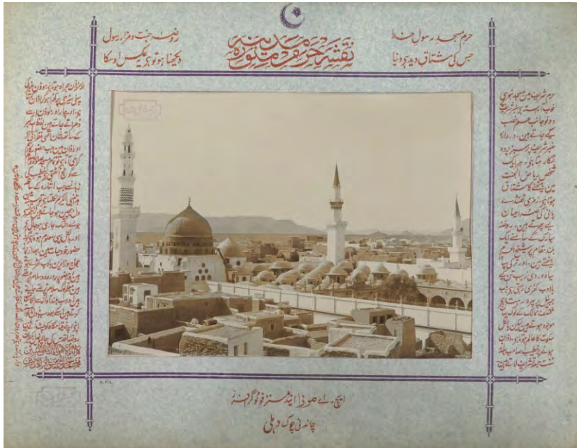
FIGURE 8.1 Picture of the Sanctuary of Medina the Radiant (c. 1907)
