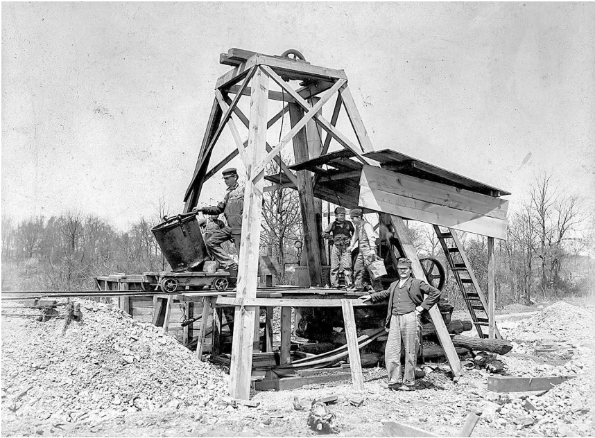
Poor man's mine, ca. 1880s. R620, 2-015. Courtesy State Historical Society of Missouri Research Center, Rolla.
