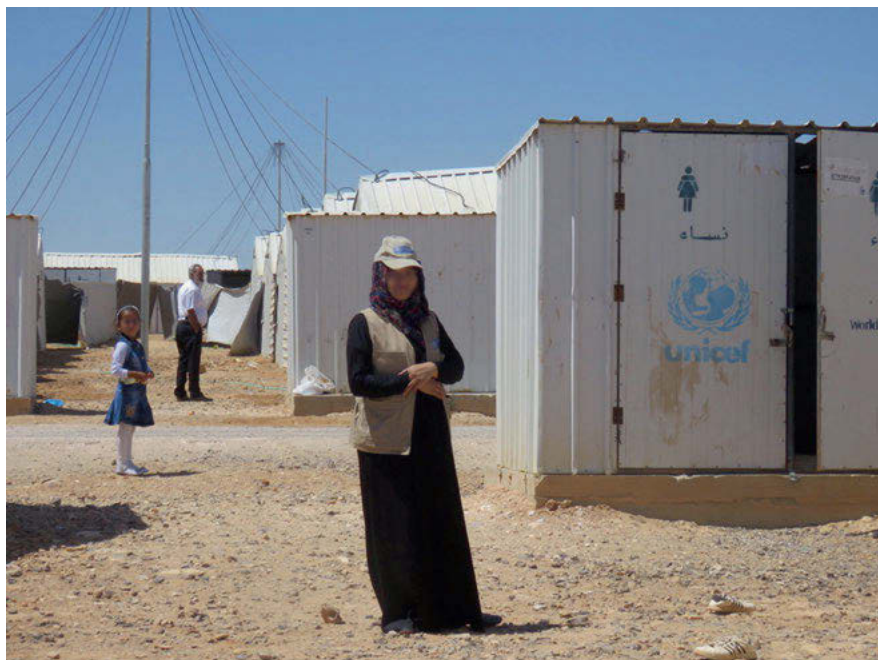
Fig. 1: The branded toilets of Azraq camp Photo: Melissa Gatter, 2018, with faces blurred out.
