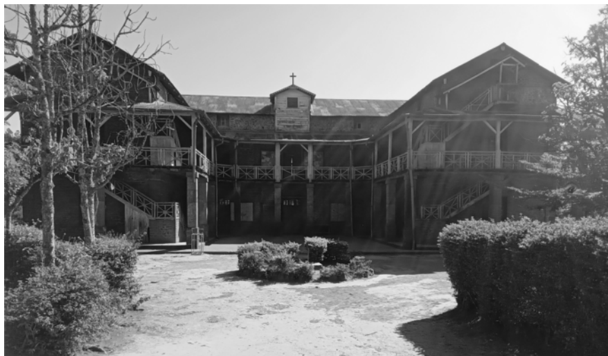
Figure 22: An abandoned German-period school at Kilema lying precariously due to seismic activities. Photographed by author, 28 th January 2023.
